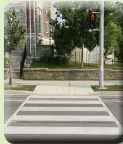
Enhanced Pedestrian Crosswalk Markings
