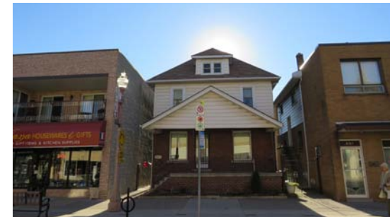
Figure 148. A residential dwelling nestled between two Main Street type buildings
