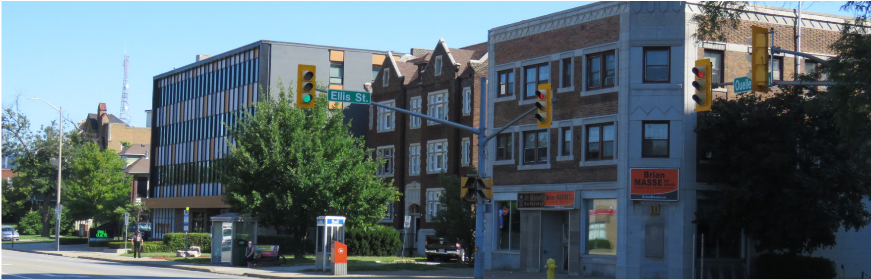
Figure 166. Inconsistent setbacks and building heights exist along Ouellette Avenue
