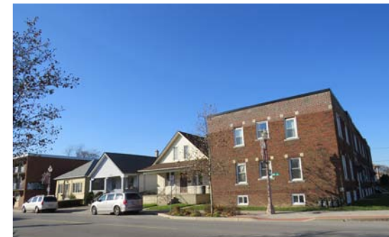
Figure 149. Residential buildings fronting onto Erie Street East, at Pierre Avenue intersection
