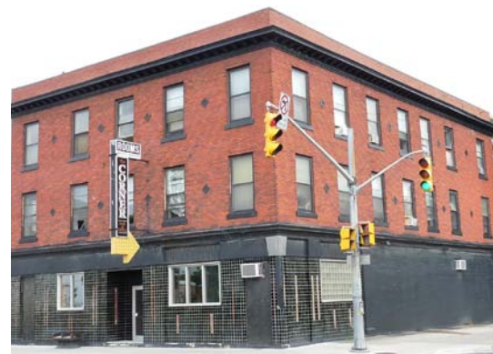
Figure 80. Wyandotte Street E, Windsor
