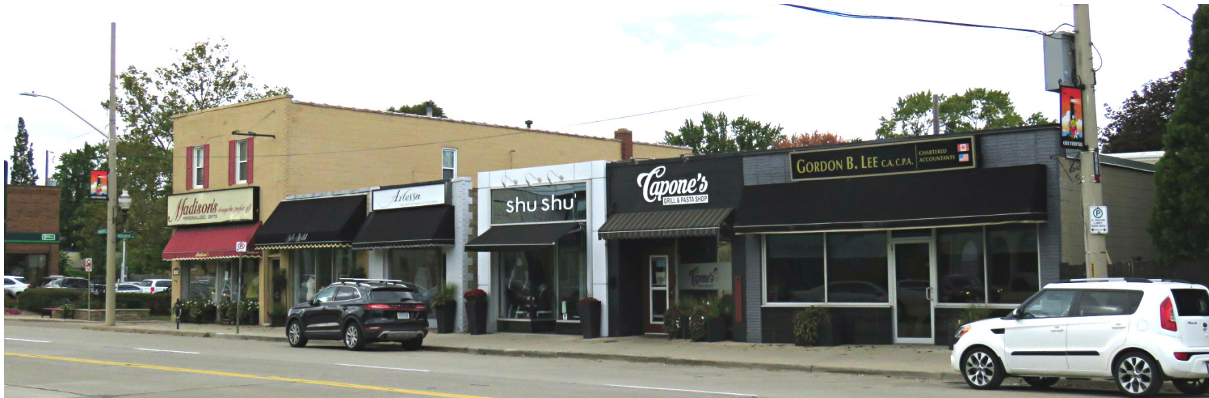
Figure 131. Building façades along the north side of Wyandotte Street East in the Olde Riverside Town Centre BIA
