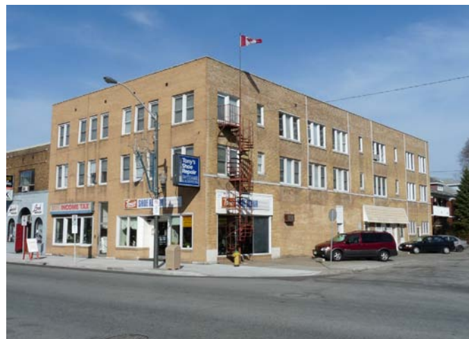
Figure 74. Leatherdale Block located at 1380-1394 Wyandotte Street East
