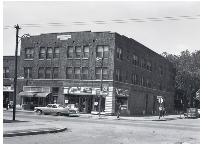
Figure 73. Leatherdale Block located at 1380-1394 Wyandotte Street East (1960)
