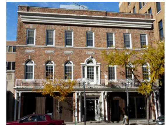
Figure 49. Equity Chambers building retains traditional brick cladding and architectural details
