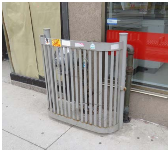
Figure 39. Site mechanical equipment at rear if possible instead of along the front facade
