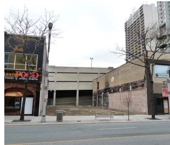
Figure 41. Avoid large breaks in the street wall such as this example along Ouellette Avenue
