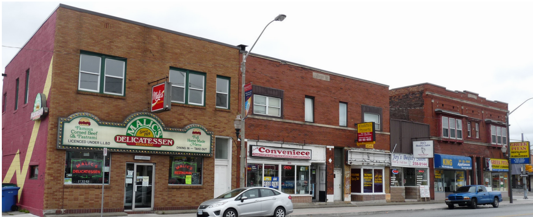
Figure 42. All store fronts are unique and are clearly distinctive through building material and architectural features
