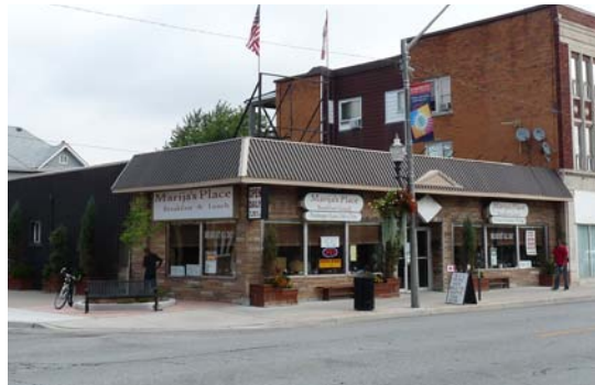
Figure 75. 1412 Wyandotte Street East
