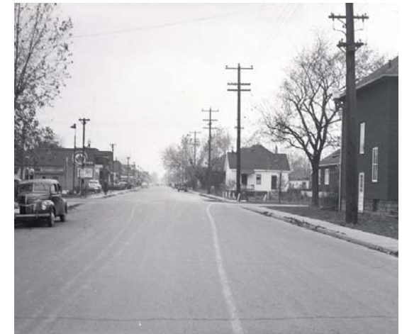
Figure 140. Erie Street East looking west from Gladstone Avenue, October 1951
