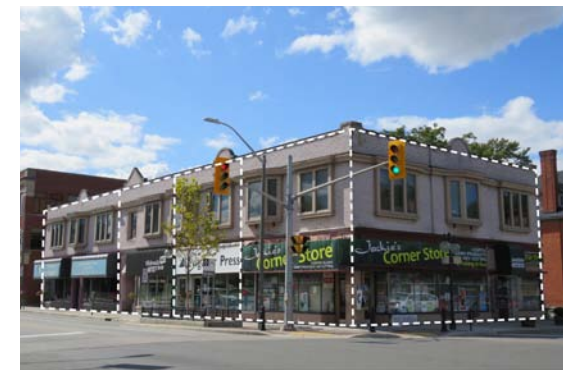
Figure 16. Strathcona Building with several storefronts identified for the purpose of the program (Walkerville BIA)
