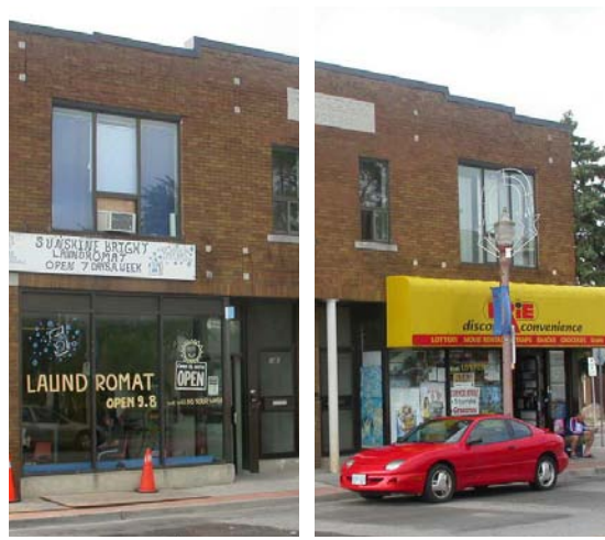
Figure 37. Window on the left is open whereas on the right it is blocked with signs
