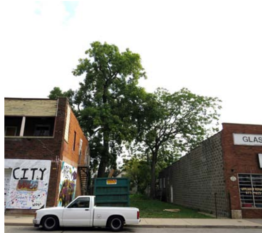
Figure 107. Gap in the street facade along Drouillard Road, Ford City, Windsor
