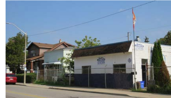
Figure 112. Example of a hodge-podge of building types and materials on the east side of Drouillard Road north of Metcalfe Street
