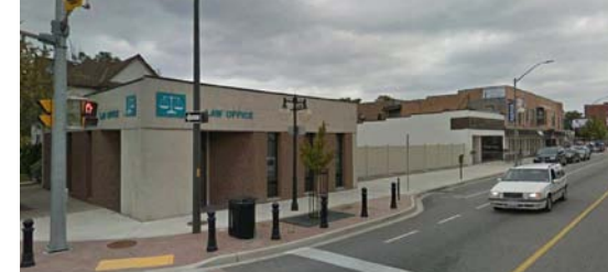
Figure 93. Wyandotte Street East between Lincoln Road and Windermere Road. Missing storefronts and inconsistent building heights and styles weaken the traditional main street.
