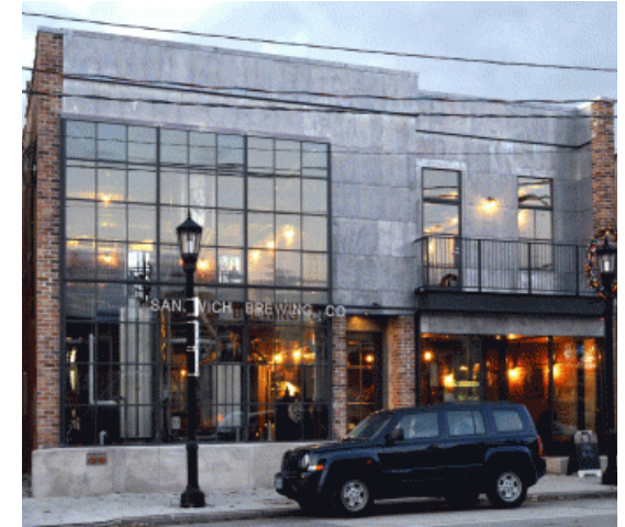
Figure 58. 3236 Sandwich Street at completion
