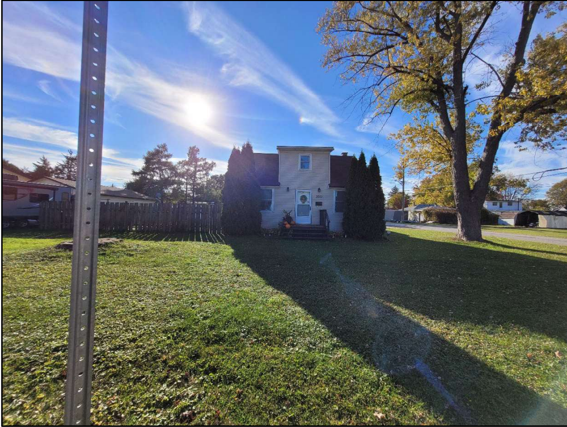
Figure 1b – Street View, from Byng Road (Source: Pillon Abbs Inc.)
