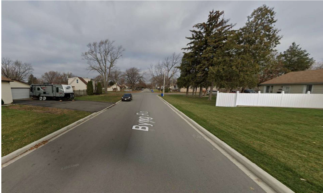
Figure 1: Looking North on Byng Road toward Lappan Avenue
