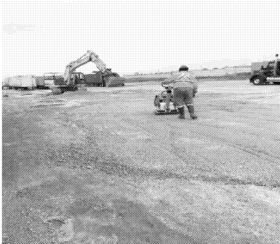
Photograph 13: placing and compacting backfill (02/10/19)
