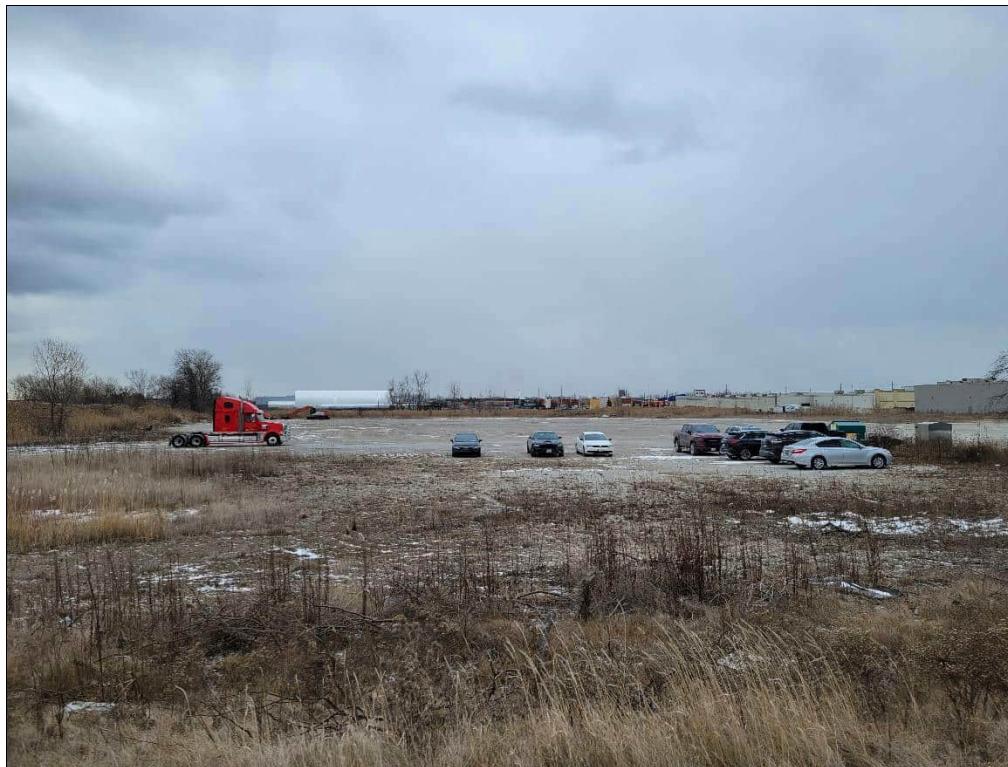
Photo 14: General overview of 2415 Division Road. Photograph taken next to the office building.
