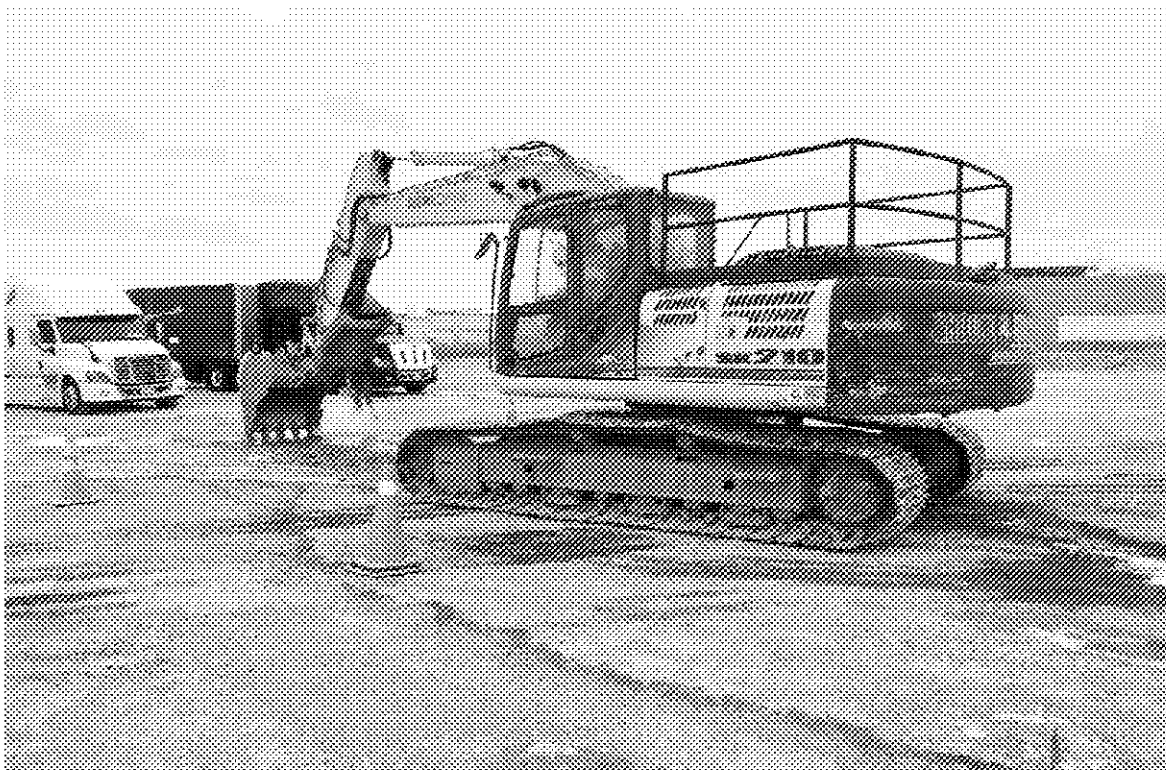
Photograph 8: excavation of impact zone (02/10/19)
