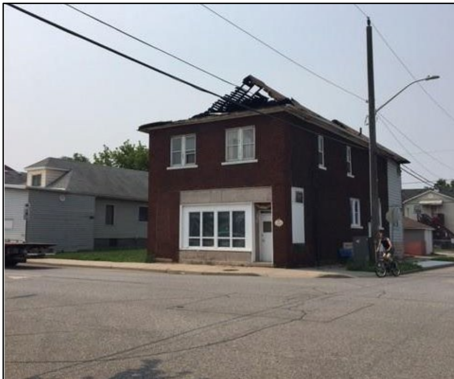
Figure 1d – Street Photo (Source: Google Earth, 2025)
