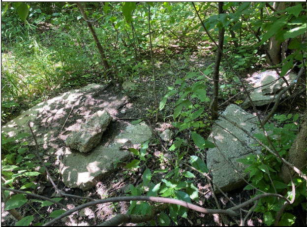
15. Partially buried concrete slabs.
