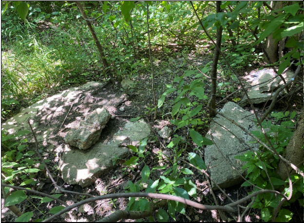
15. Partially buried concrete slabs.
