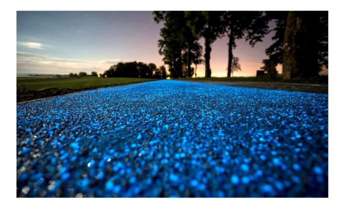
Although the Starry Night bike path provided inspiration, the technology used in producing the Polish bike path differs slightly. Studio Roosegaarde used LED lamps, solar panels, and "light-accumulating paint." The bike path designed by TPA Sp. z o.o. does not require any alternative power sources. The path is still being tested to gather information about its wear and durability.
