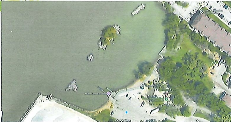
Mckee Park Shore works
