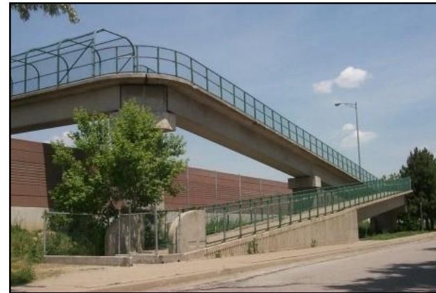
Photo: E.C. Row Expressway overpass at Mark Avenue – Windsor, Ontario
