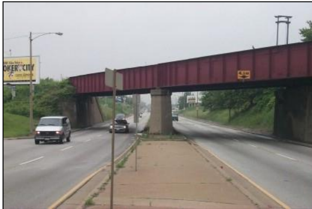
Photo: Rail underpass on Dougall Avenue – Windsor, Ontario
