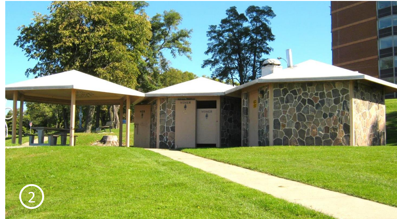
EXISTING WASHROOM BUILDING
