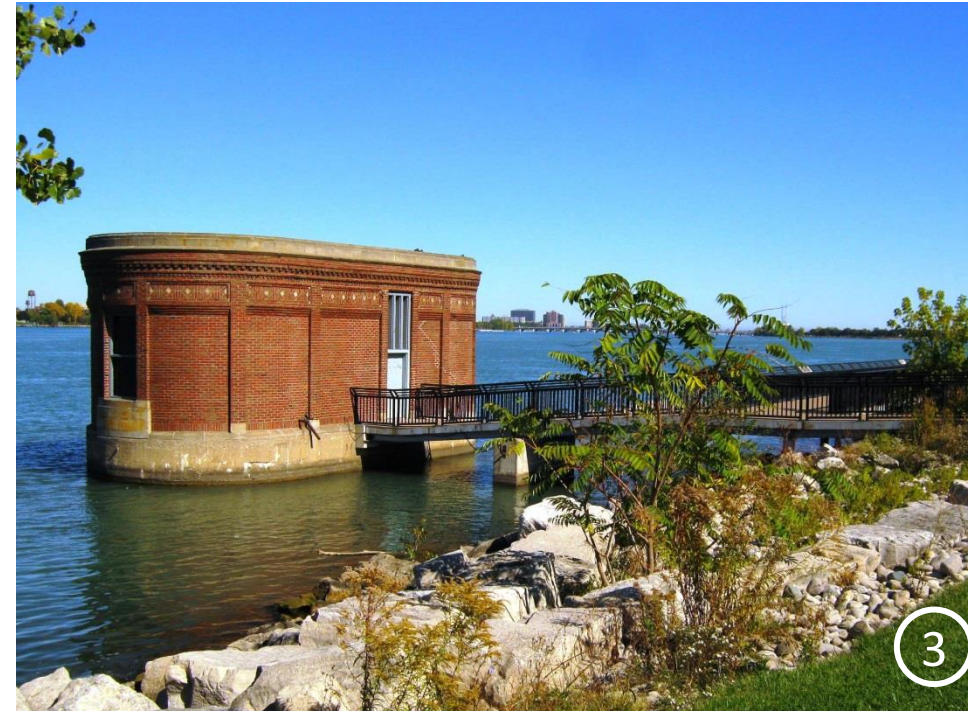
PUMP HOUSE (DAWN BEACON)
