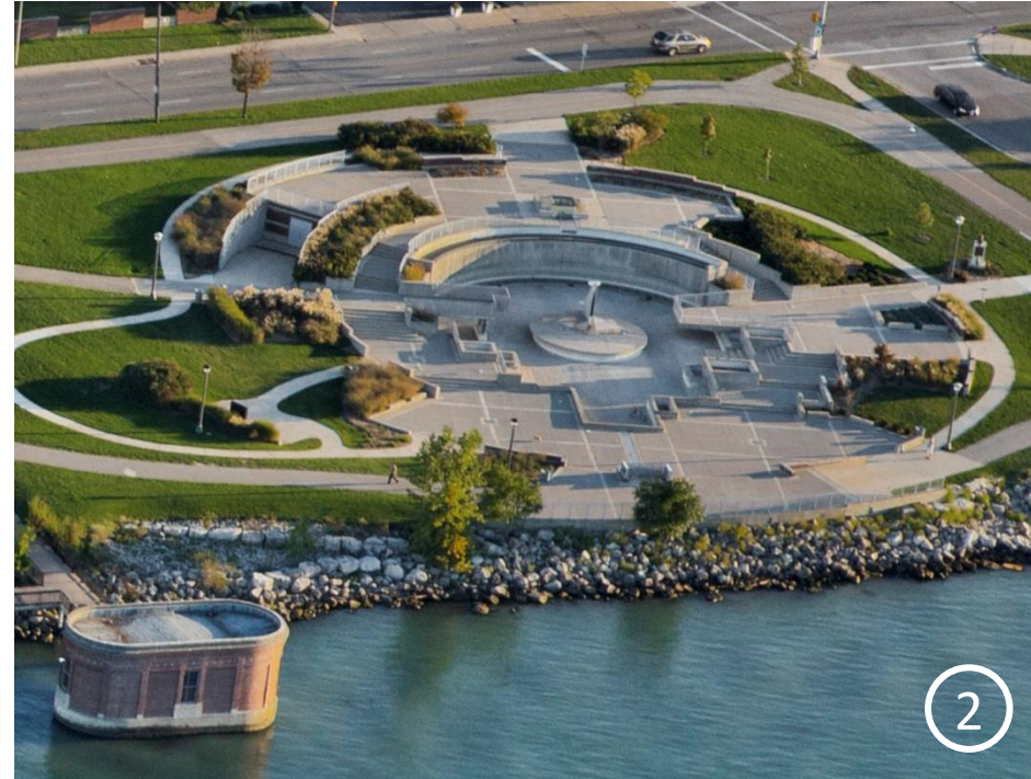
FOUNTAIN AND PUMP HOUSE
