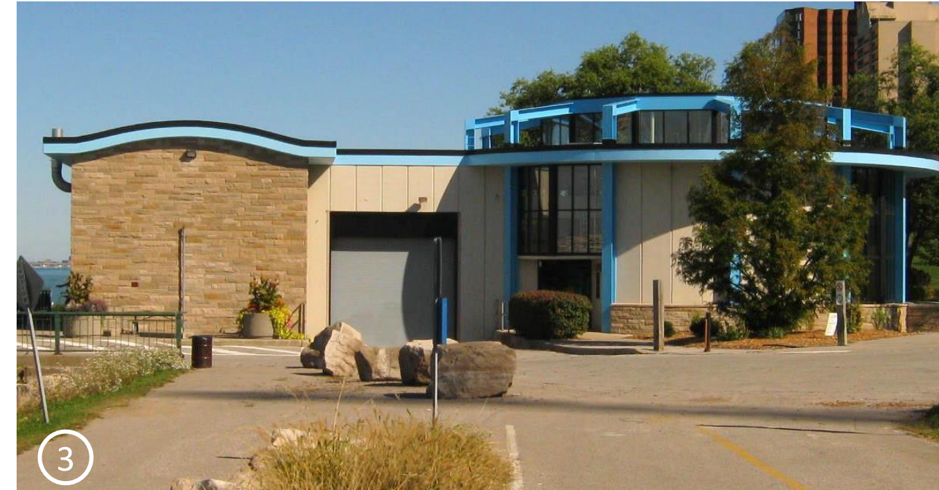
CARON AVENUE PUMP STATION
