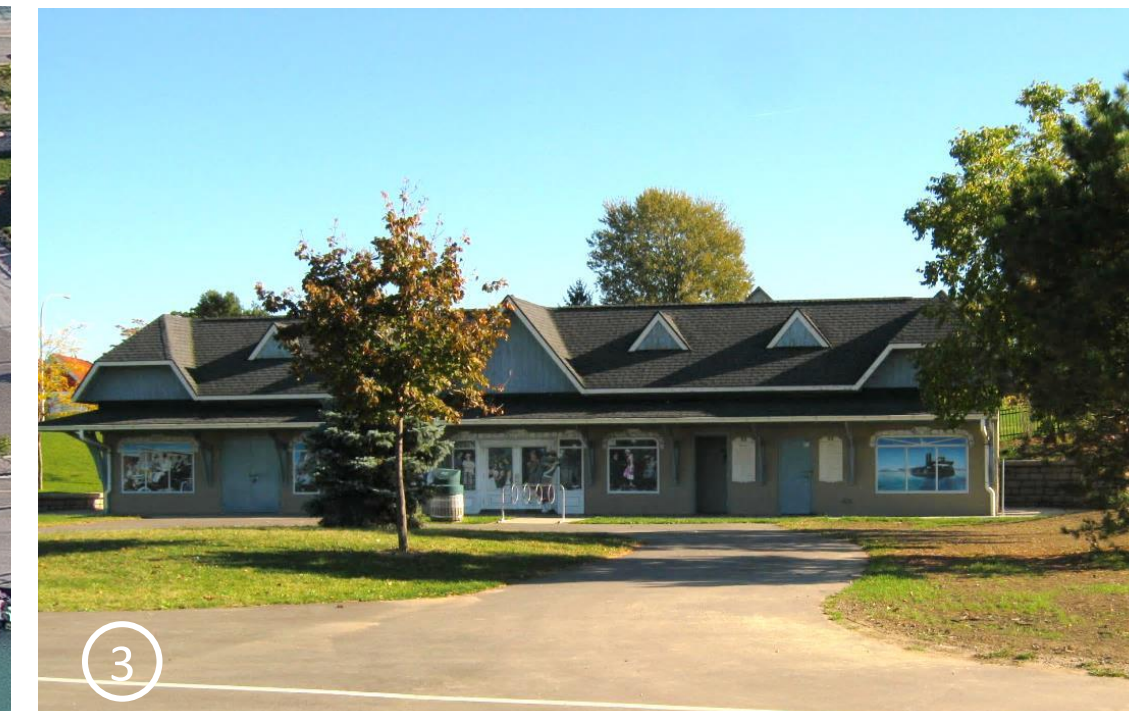
WASHROOM AND MAINTENANCE BUILDING
