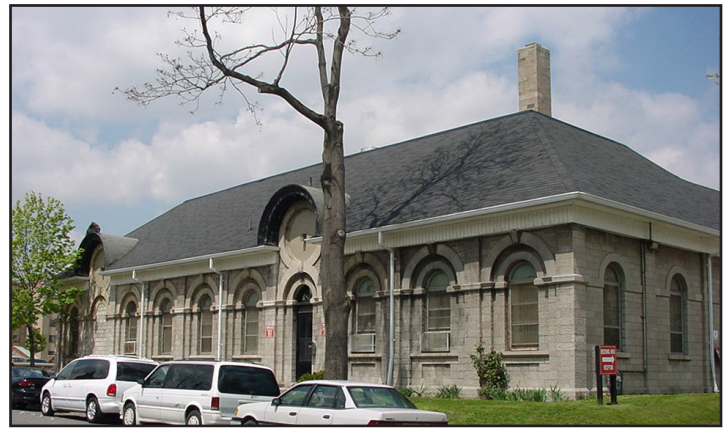
Brock Street Registry, a landmark listed heritage property located in Olde Sandwich Towne.
