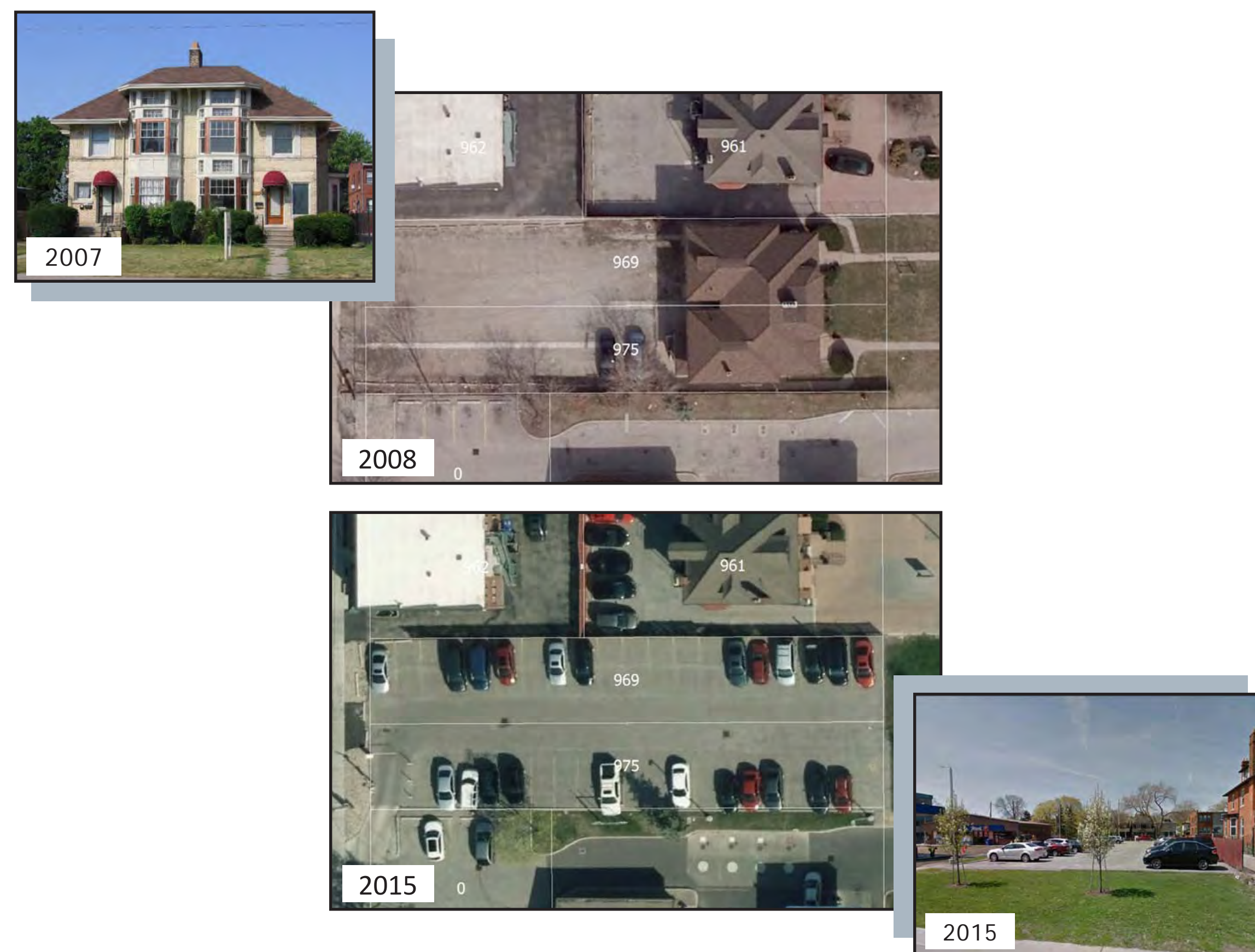
969-975 Ouellette Avenue, demolished in 2009. An example of a residential building demolished for parking.
