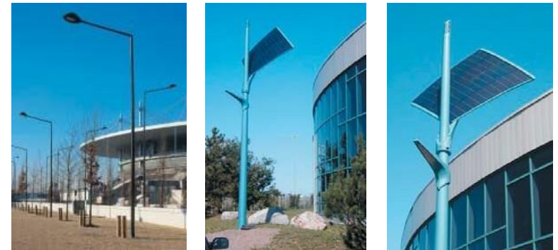
Examples of lighting standards and the incorporation of photovoltaic panels
