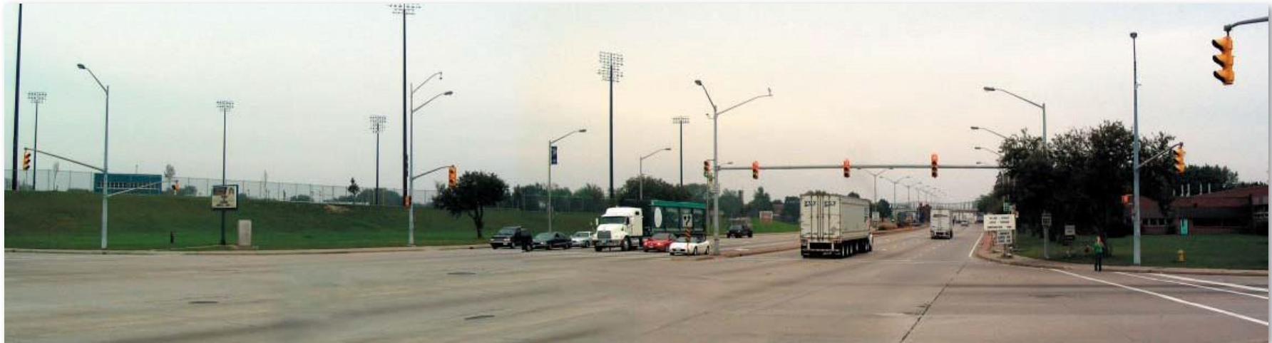
EXISTING CONDITIONS AT HURON CHURCH RD AND COLLEGE AVE LOOKING SOUTH
