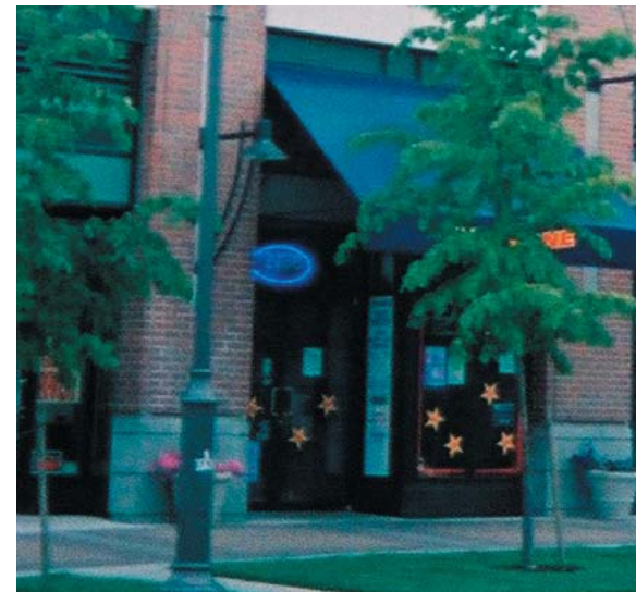
At grade entranceways with overhangs are recommended
