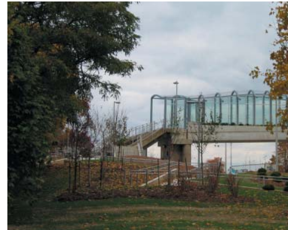
Existing earthwork berm at 'Green Bridge' on Huron Church
