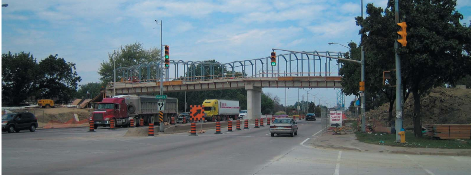
View of Green Pedestrian Bridge during construction
