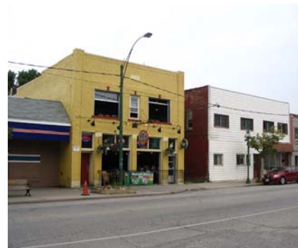
Existing built form along Sandwich Street.
