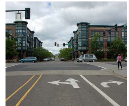
Major intersections should have paved crosswalks that are highly visible by oncoming traffic.
