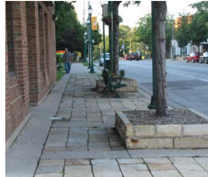
The limestone pavers used through Sandwich Street should be continued to the Detroit and Sandwich Street intersection.
