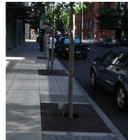
In areas along the public walkway where there is insufficient room for a raised planter, sunken structural soil pits with tree grates are recommended.
