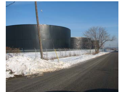
Storage tanks and typical street edge condition along Russell Street within the Industrial Area.
