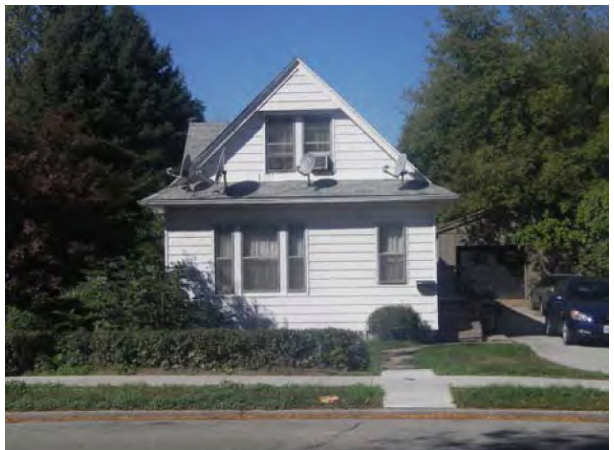
The numerous satellite dishes populating this building provide visual clutter.
