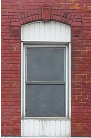
A vinyl-infilled window on the J. Spiers Building.
