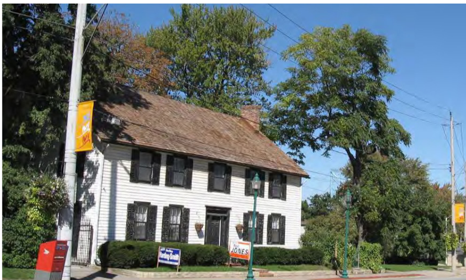
The MacGregor-Cowan House is surrounded by trees that are over a century old and provide invaluable landscape context to the home.
