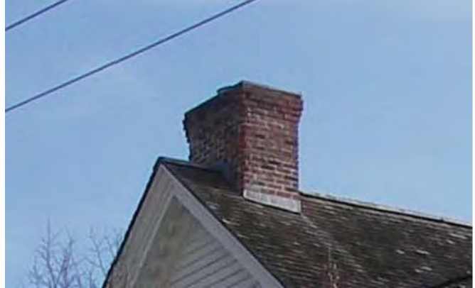
A typical brick chimney with original corbelling.
