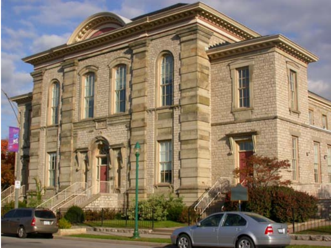
Mackenzie Hall, an important built element within the Sandwich streetscape.
