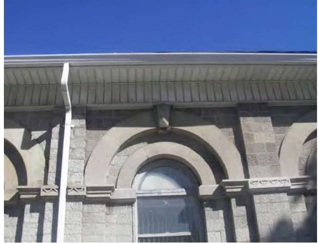
The eaves trough on the Registry Office cuts through the stone detailing of the façade. This damage is both regrettable and irreversible.
