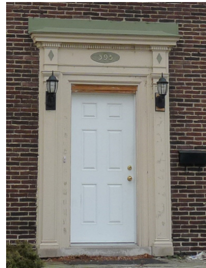
A classically treated door at 395 Rosedale Avenue.
