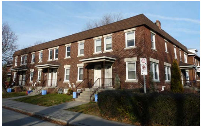
376-386 Rosedale Avenue. This building respects both the massing and setback of the surrounding building stock.
