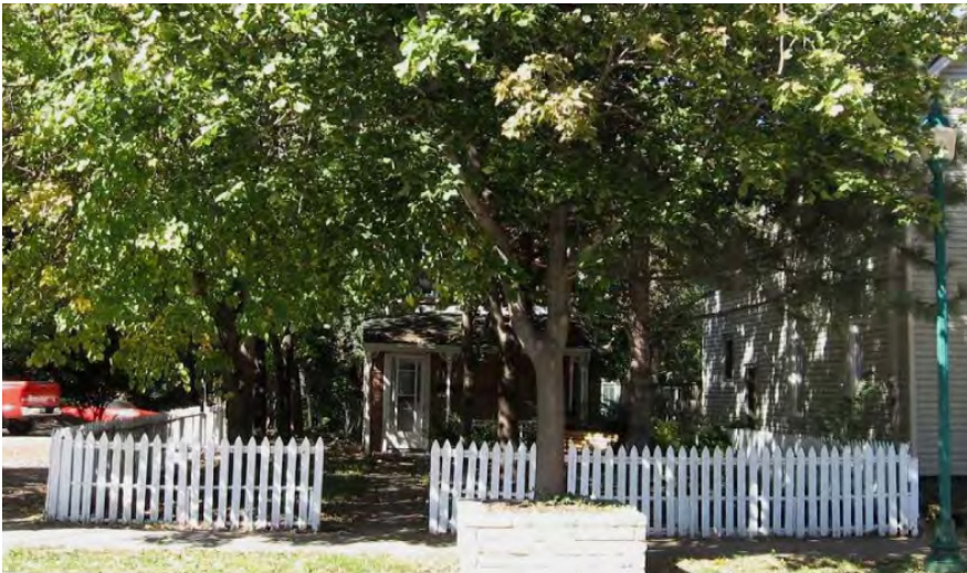
A former picket fence at 3164 Sandwich Street served to separate public from private, and define the landscape
