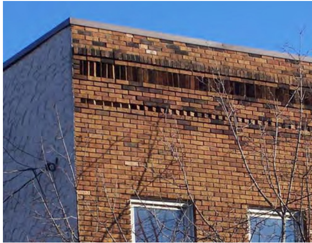
Commercial brick work from ages past.
