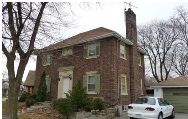
395 Rosedale Avenue. Note the Georgian Revival elements and sensitivity to the streetscape.
