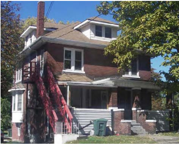
An unsympathetic exterior fire staircase.
