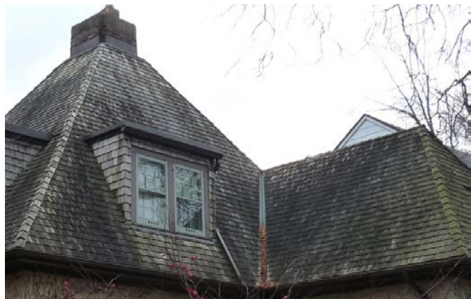
Cedar shingles on the Masson-Deck house.
