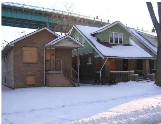
Boarded up houses on Indian Road
