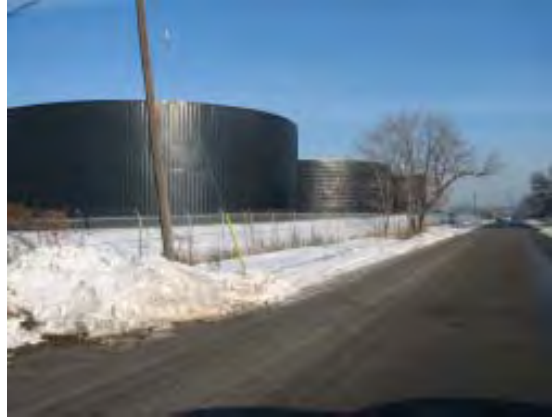
Fuel Storage Facility on Russell Street
