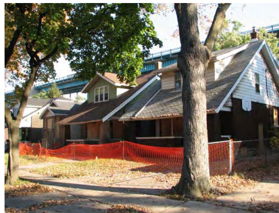
Boarded up houses on Indian Road
