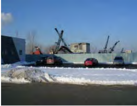
Metals Recycling Facility on Russell Street
