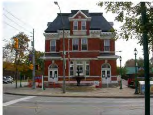
3201 Sandwich Street (Post Office)
