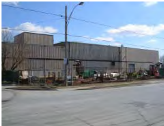
Industrial building with outside storage at southeast corner of Sandwich Street and Prince Road
