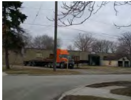
Rear of industrial building at southwest corner of Hill Avenue and Peter Street
