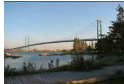
Extending the riverwalk into the Sandwich Area has previously been identified as an important City initiative and would provide a direct connection from the central city to Olde Sandwich Towne's waterfront and main street
