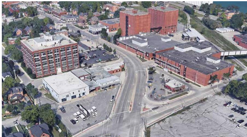
Figure 100. Bird's Eye View - Existing Condition
