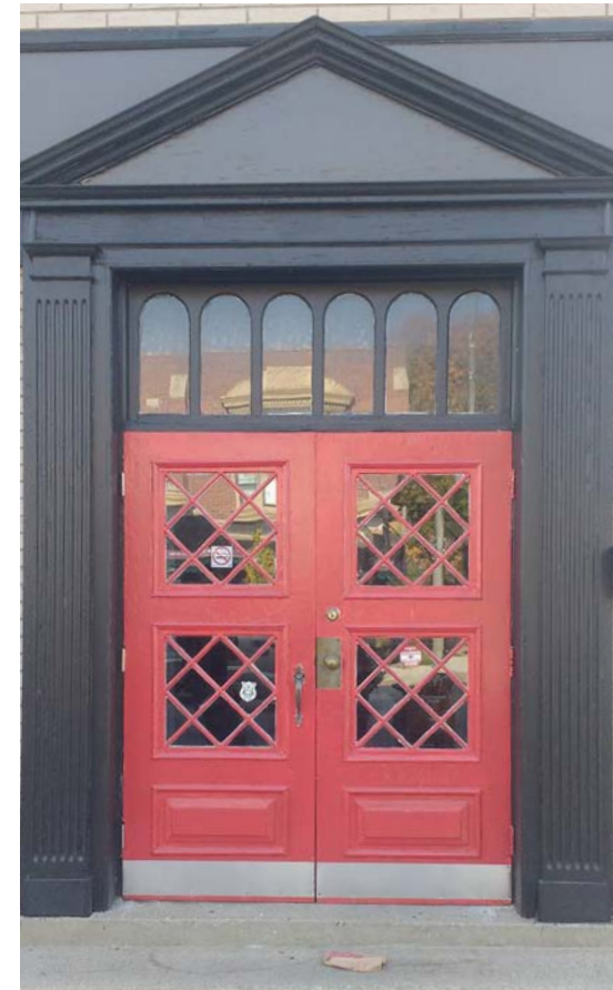
Figure 55. Distinct doors can make a business more visible and improve the overall appearance of the storefront
