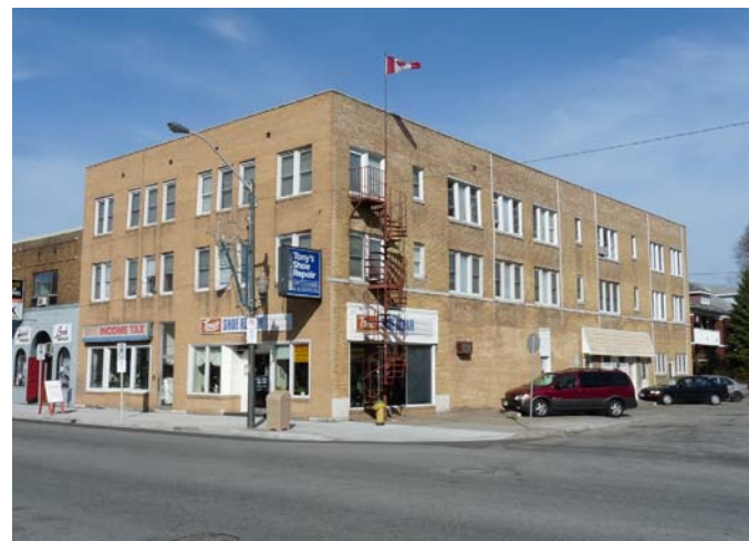
Figure 74. Leatherdale Block located at 1380-1394 Wyandotte Street East
