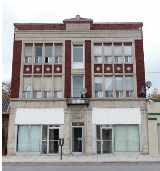
Figure 77. Pasadena Block located at 1424-1434 Wyandotte Street East
