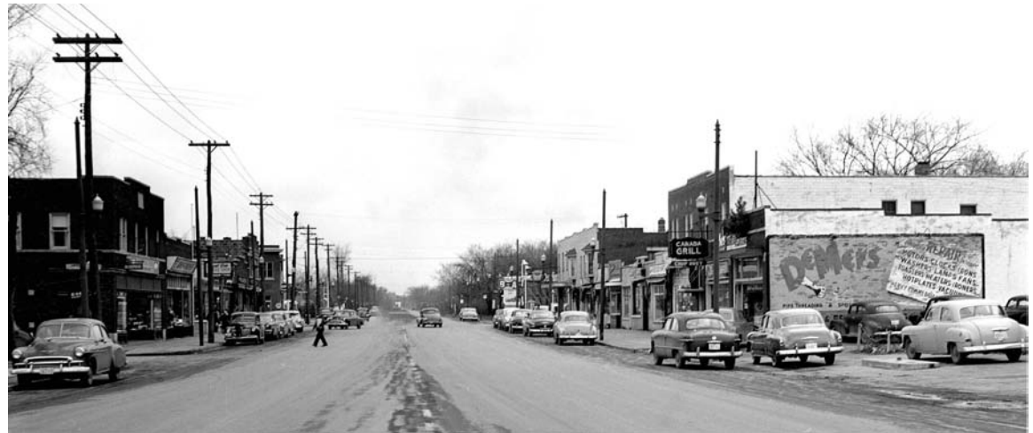
Figure 115. Wyandotte Street East, looking west from Lawrence Road, December 1952 (Edwards and Weeks)
