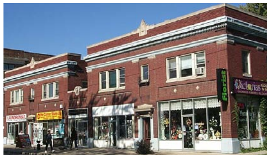
Figure 45. Traditional Main Street building on Erie Street W
