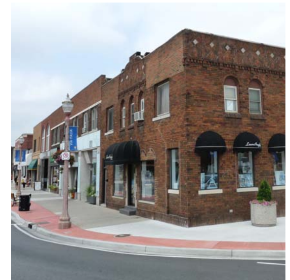
Figure 20. Erie Street and Parent Avenue, Windsor
