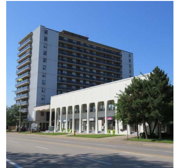
Figure 167. Example of an International Style building
