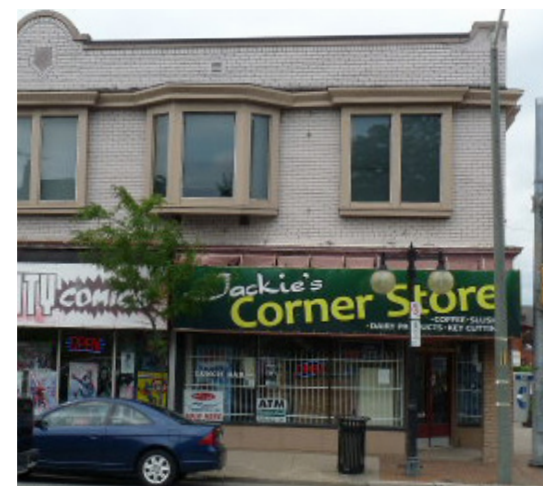
Figure 89. Security bars on windows make the area feel unsafe
