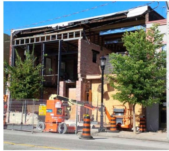
Figure 57. 3236 Sandwich Street during renovations
