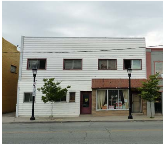
Figure 56. 3236 Sandwich Street before renovations, 2012
