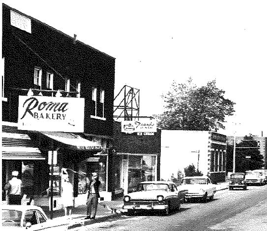
Figure 129 Traditional Main Street facades along Wyandotte Street East by St. Louis Avenue, date unknown (Fullerton)
