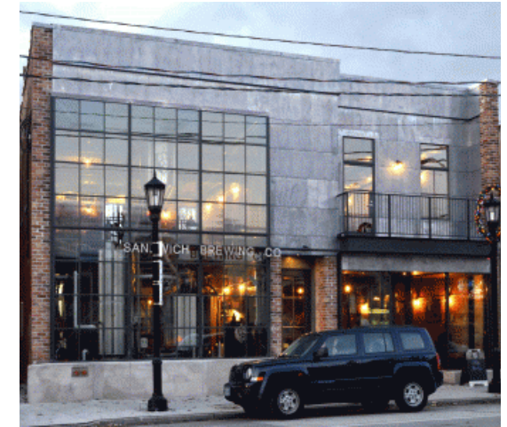
Figure 58. 3236 Sandwich Street at completion
