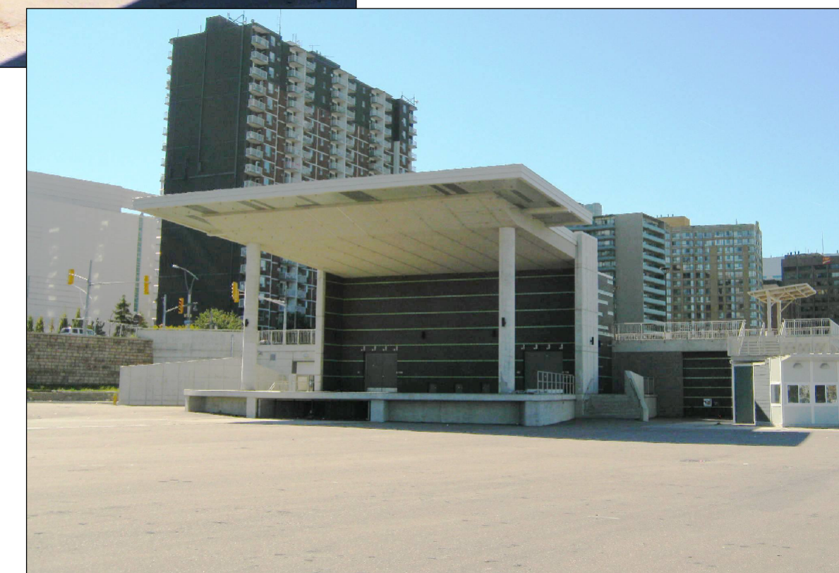
EXISTING SITE – LOOKING SOUTH WEST FROM RIVERWALK
