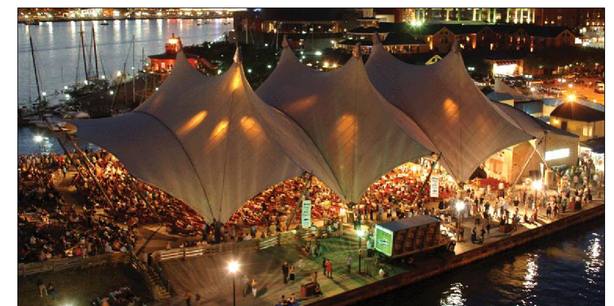
ROOF STRUCTURE/CANOPY OVER CONCERT SEATING AREA
