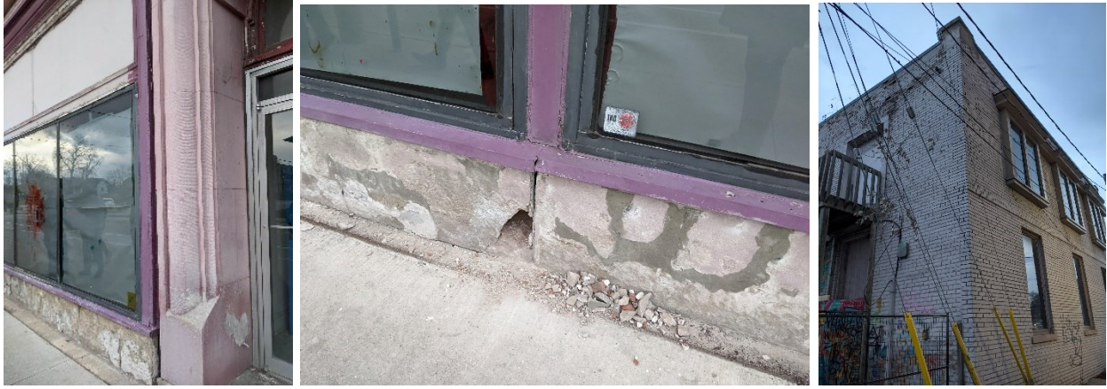
Photographs of the building in its previous state, showing some deterioration of storefronts
