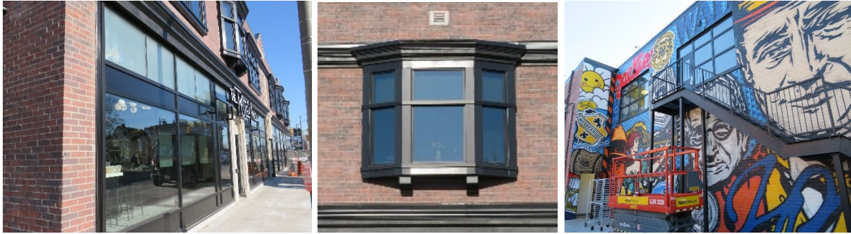
Restoration work conducted and the finished building
