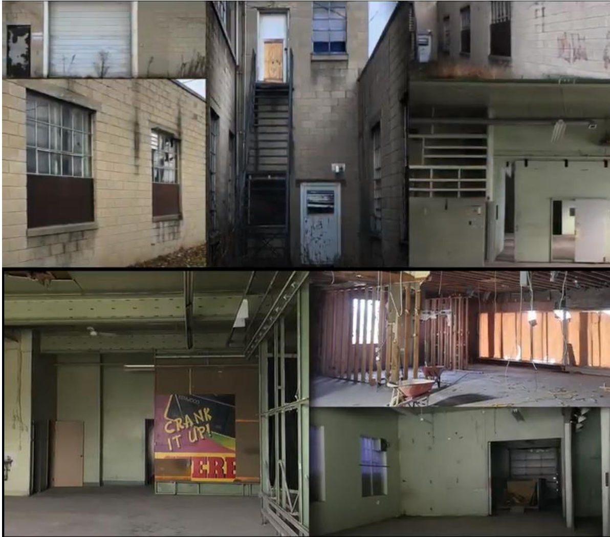
Pre-renovation photos. (Source: Lester Group).
