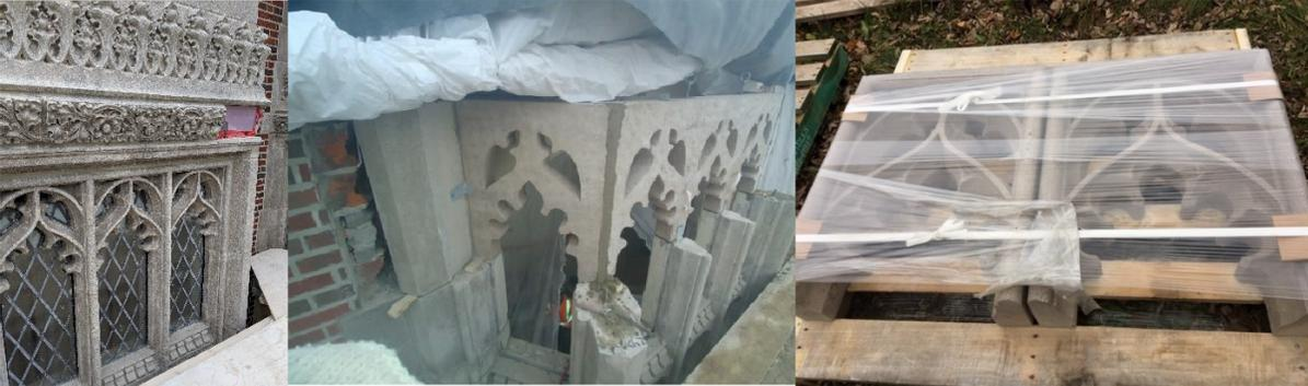
Inspection of underlying steel structure, removal and shipping of precast stone at oriel tracery for repairs
