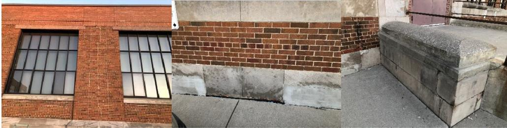
(Left) Cracking of masonry at gymnasium; (Right) Typical sections of stone/brick at base needing replacement/repair, and cleaning.
