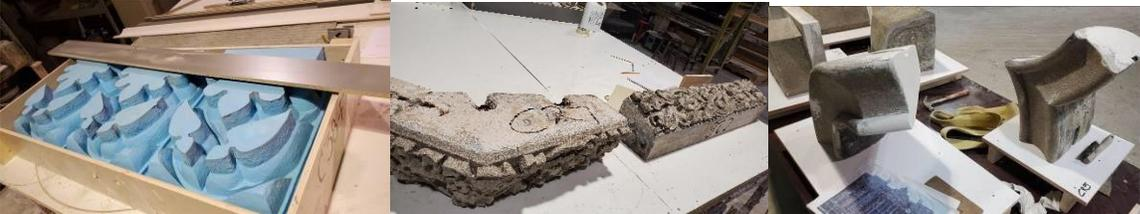
Recasting precast stone using moulds of original pieces for repairs/replacement
