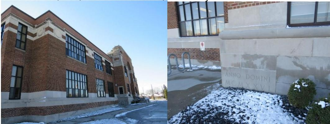
Results of the extensive repairs of masonry sections (stone and brick) at base all around the building
