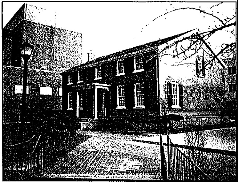
North elevation of the Francois Baby House, which faces toward the Detroit River
