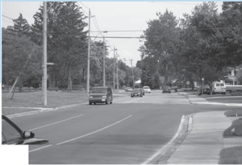
EXISTING CONDITIONS AT ST. ROSE AVENUE AND RIVERSIDE DRIVE LOOKING EAST
