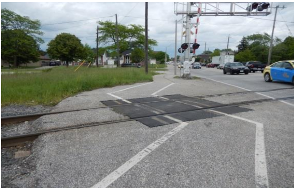
Photo 6: Sidewalk at rail crossing
