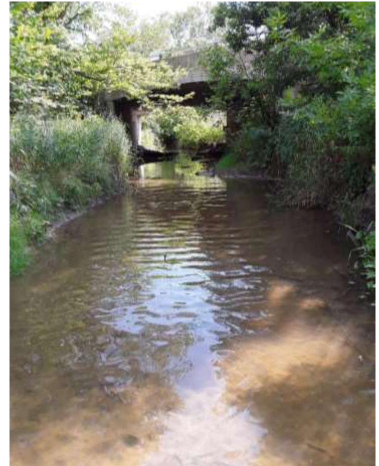
Little River Drain
