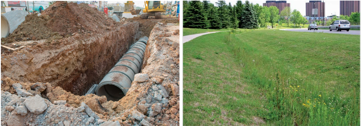
Figure 2: Storm Sewer Network (L) and Open Drain (R) Sample Images
