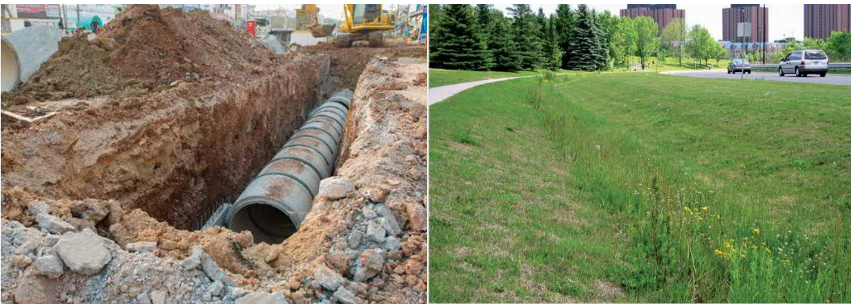
Figure 5-2: Storm Sewer Network (L) and Open Drain (R) Sample Images
