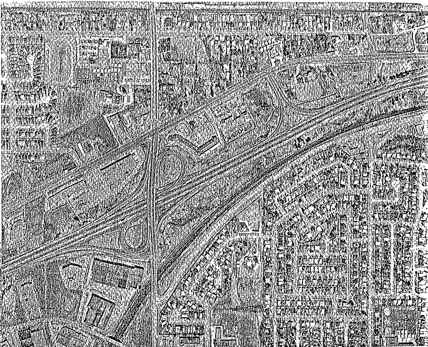
Figure G.3 'BUTTONHOOK' EXIT RAMP: HIGHWAY 401 - PICKERING, ONTARIO
