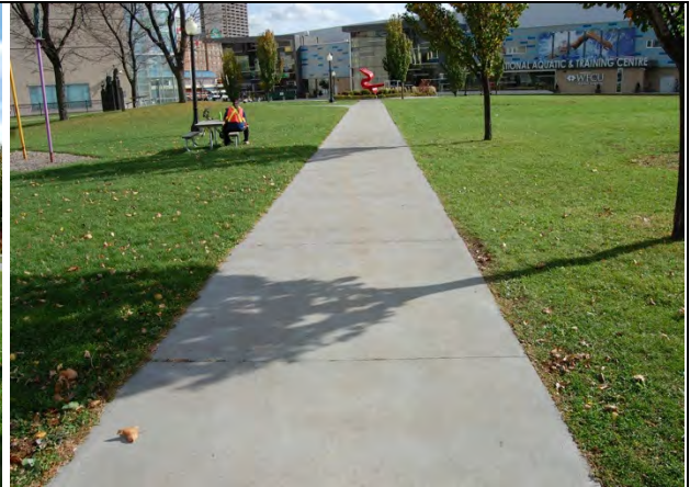
PLATE 8 SITE 1 CONCRETE WALKWAY
