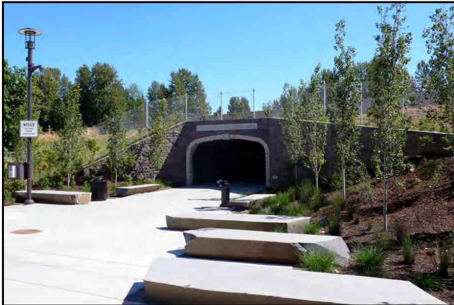
Pedestrian tunnel in Washington State features both a “flared” opening, combined with public seating areas to allow for ongoing monitoring of the tunnel space
