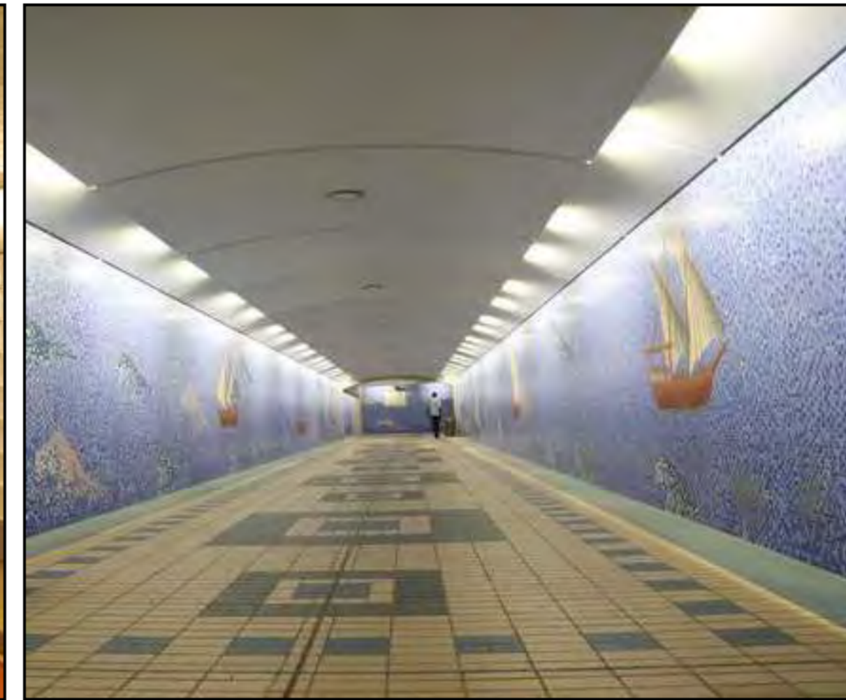
Lighting built into walls and ceilings are less susceptible to vandalism
