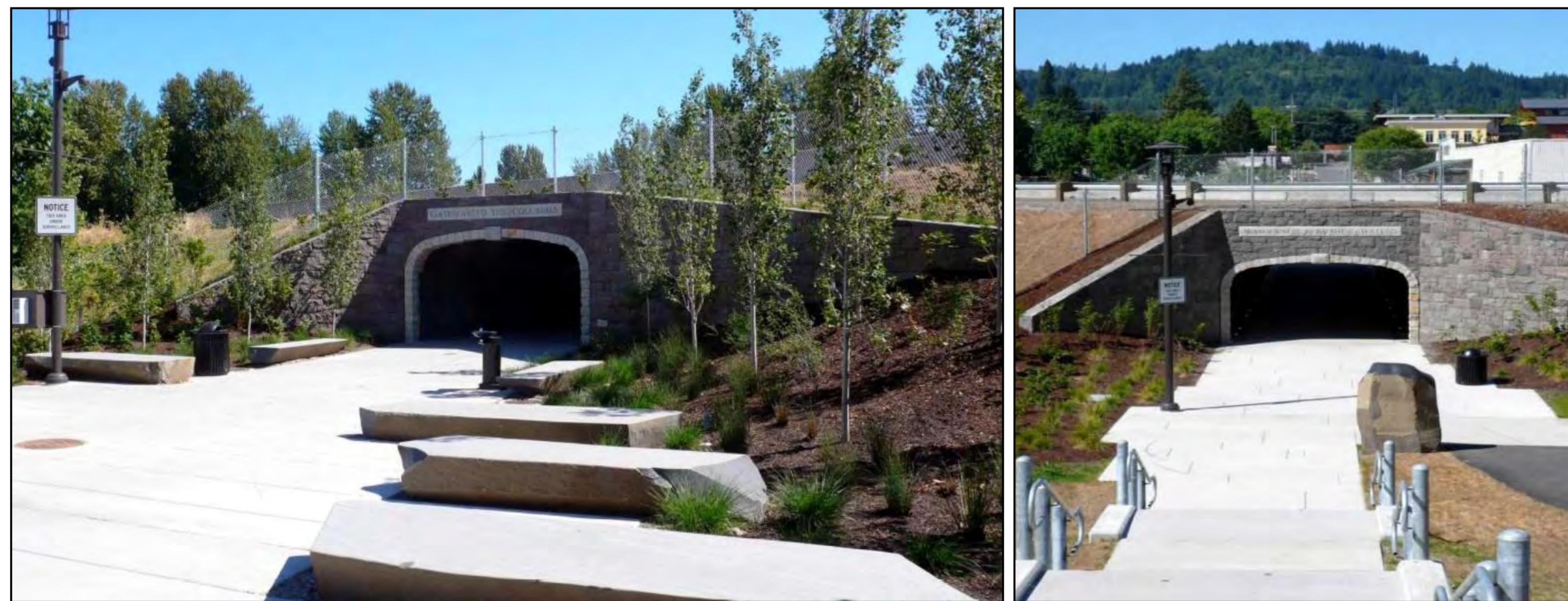
Example: Seating, flared openings and natural surveillance (gradual stairs, proper lighting and small scale landscaping elements)
