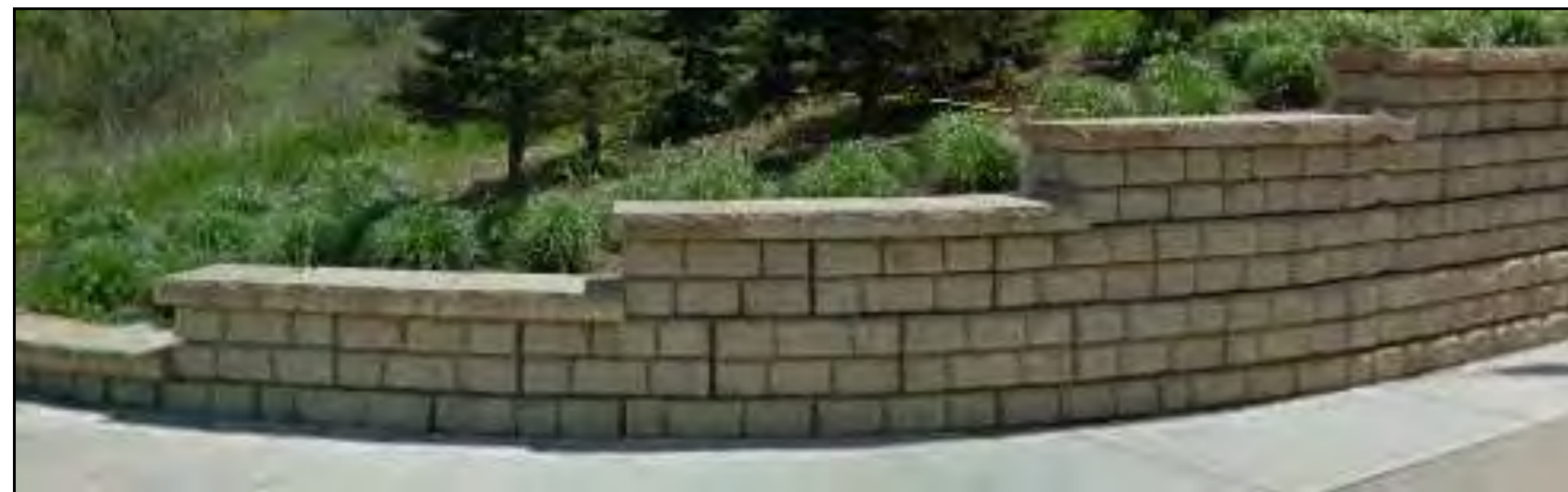
Redi-Rock retaining walls
