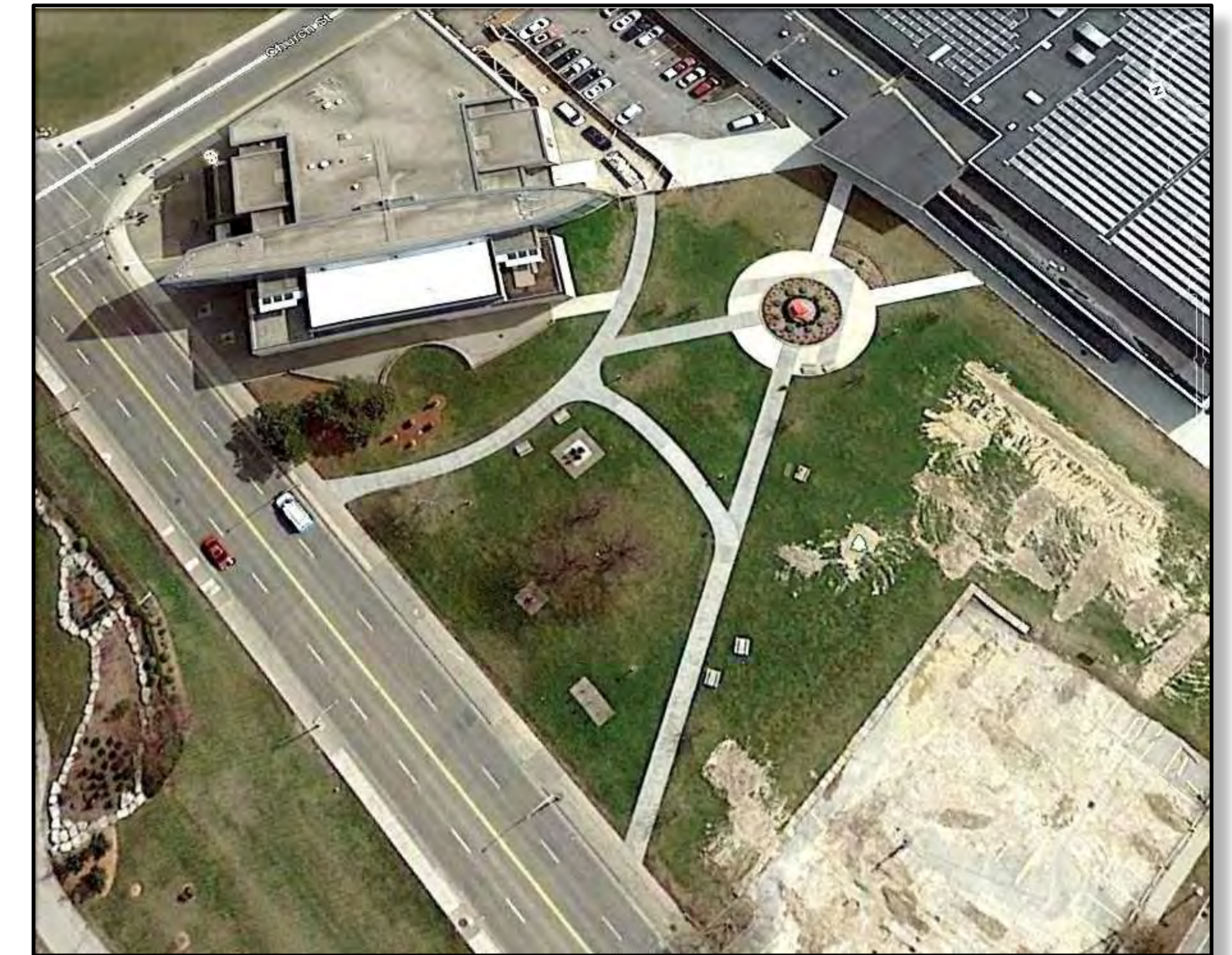
Art Gallery at Aquatic Centre Site
