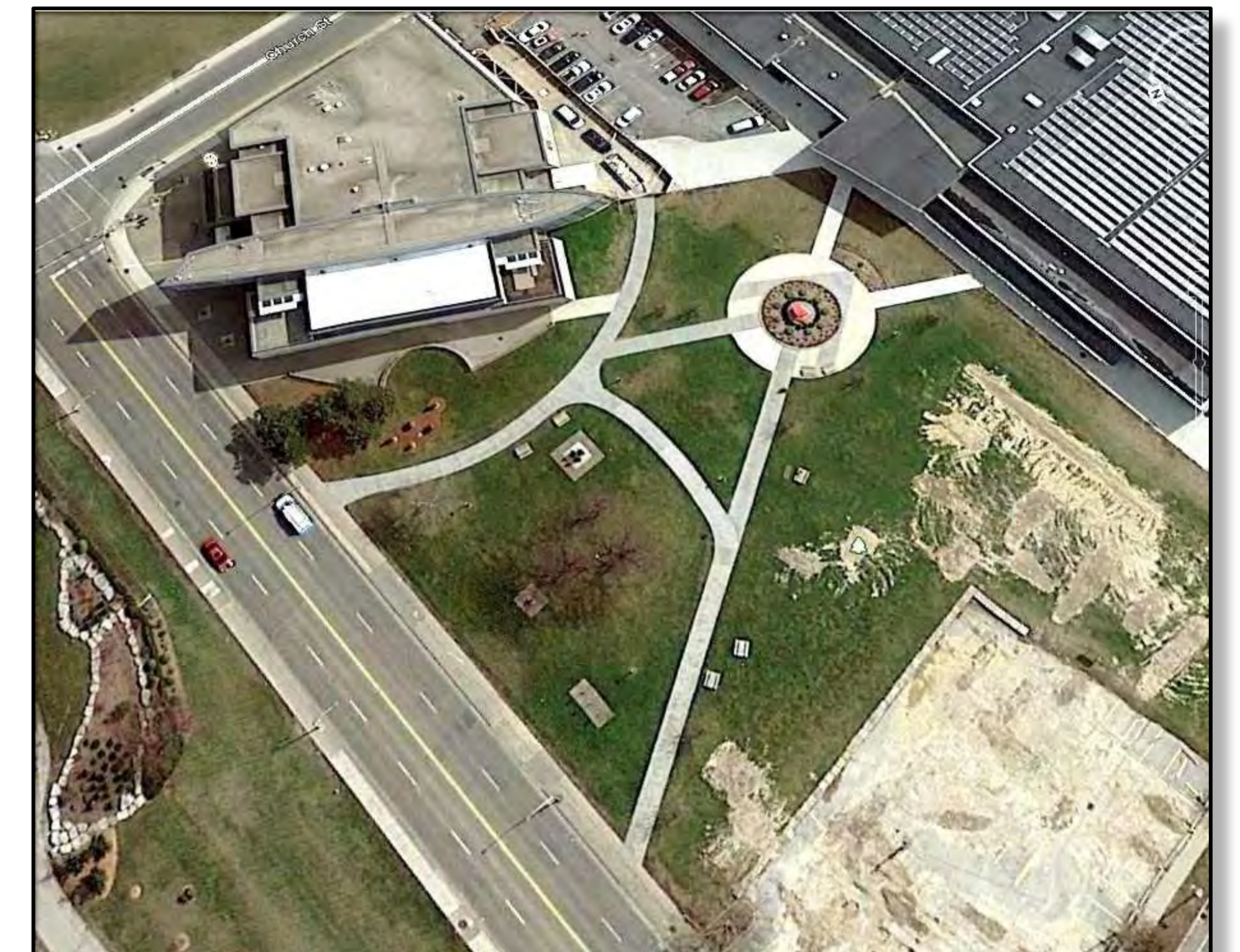
Art Gallery at Aquatic Centre Site
