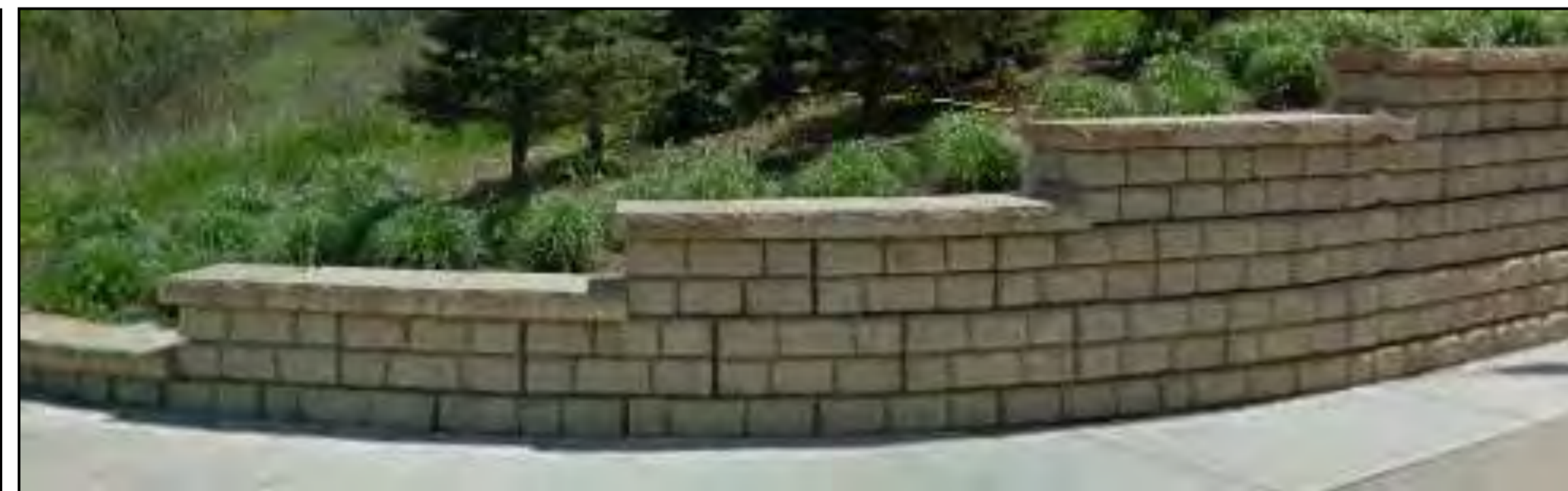
Redi-Rock retaining walls
