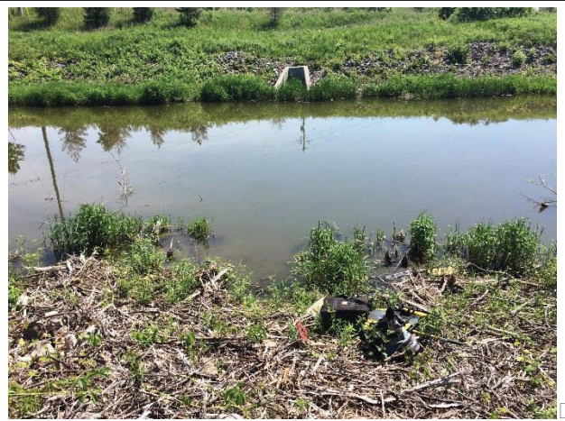
Photograph of the McHugh Street storm runoff structure
