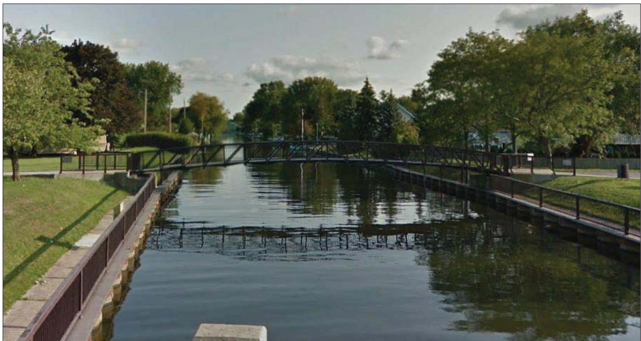
*installed downstream of Project Site on Little River
