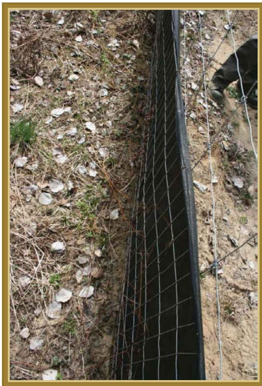
Figure 1: Exclusion mesh installed over a streambed to prevent animals from burrowing under the enclosure.
