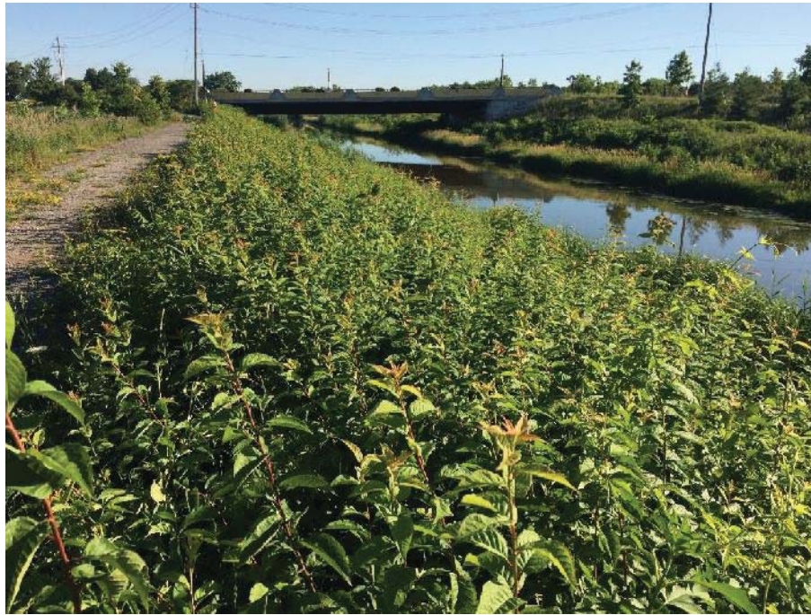
Photo 5: McHugh Bridge – West bank and pedestrian path, facing north.
