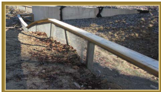
Figure 4: A wire mesh fence installed on a gravel embankment next to a road. M
