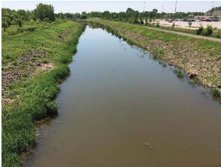
Photo 1: McHugh Bridge – Facing downstream from bridge approximately 60 m upstream.
