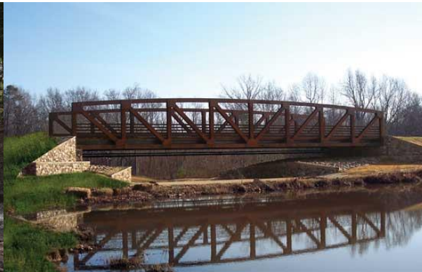
Pre-fabricated Steel Bridge
