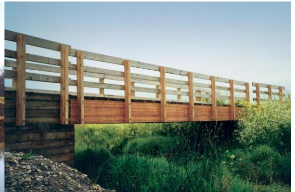
Pre-fabricated Timber Bridge
