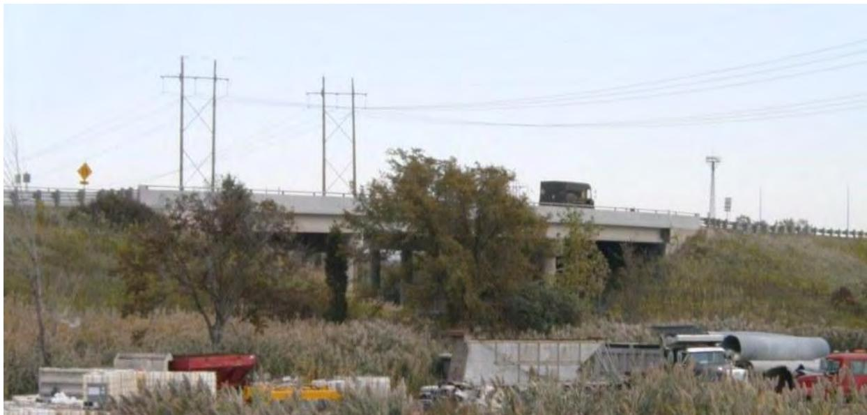
The Lauzon Parkway bridge over the Little River is located approximately 330 m north of County Road 42 built in 1981. It has a total span length and width of approximately 10.8 m and 13.1 m respectively.
