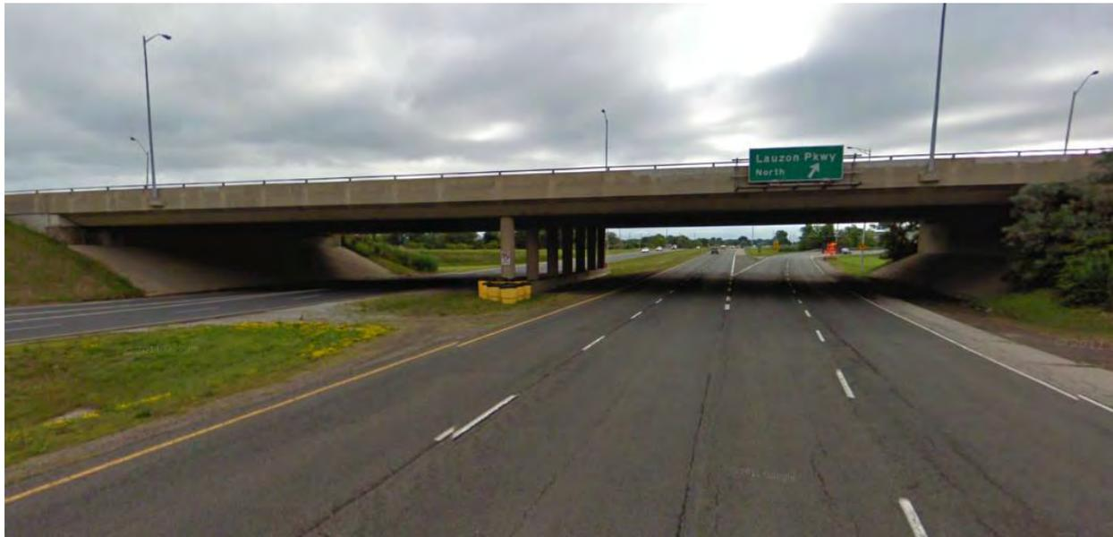
The Lauzon Parkway Bridge over the CP Rail is a 3-span pre-stressed concrete girder bridge built in 1980. It has a total span length and width of approximately 61.9 m and 24.6 m respectively. The structure was rehabilitated in 2008. Work on the structure included converting the existing abutments to semi-integral abutments and constructing new approach slabs. The structure is illustrated in Exhibit A.4-11.
