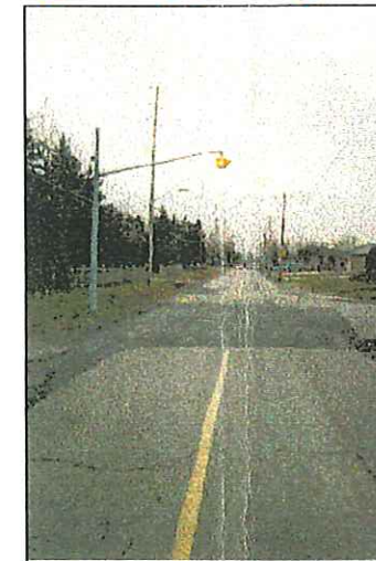
At Southdale Drive, Looking West
