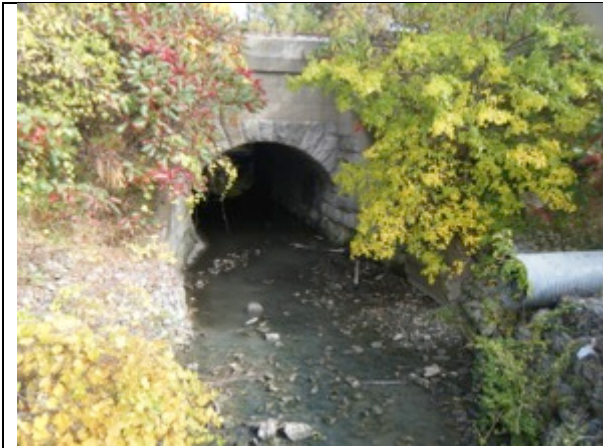
Plate 19 Drain Channel facing northeast
