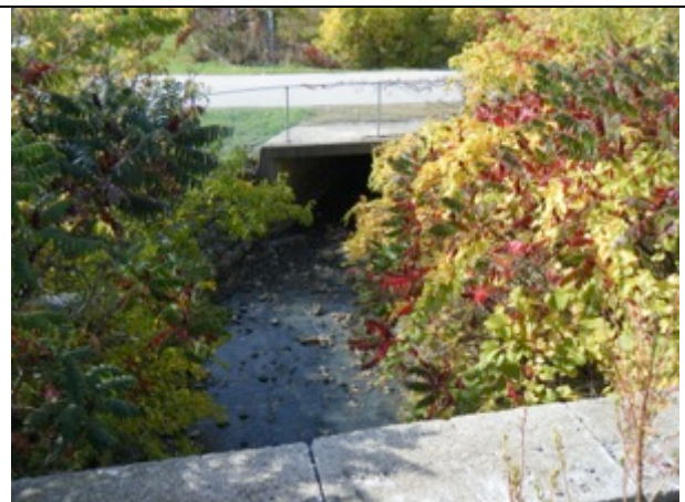
Plate 18 Drain Channel facing southwest
