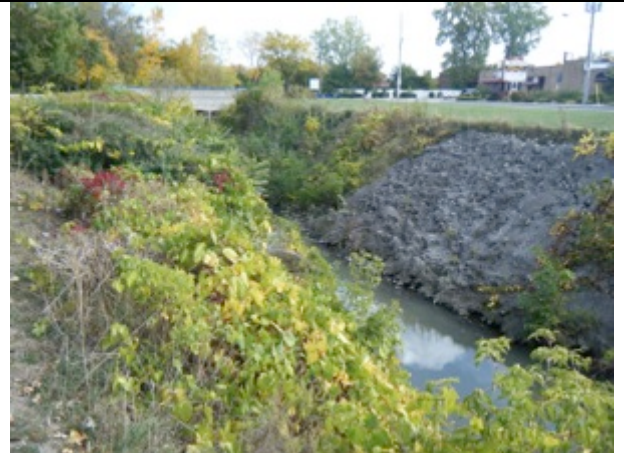
Plate 24 Drain Embankment facing northeast
