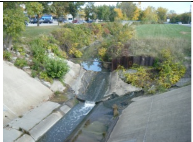
Plate 26 Drain Channel facing northeast
