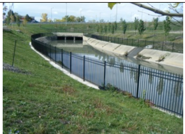
Plate 12 Drain Channel facing west
