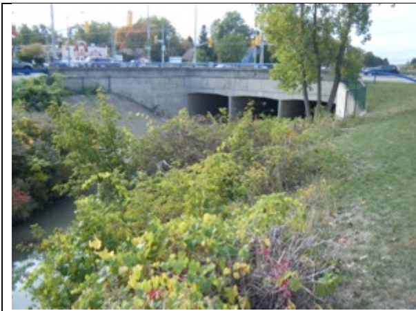
Plate 25 Drain Channel facing southwest
