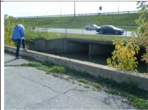
Plate 9 Entry to Passage under E. C. Row Expressway facing southeast
