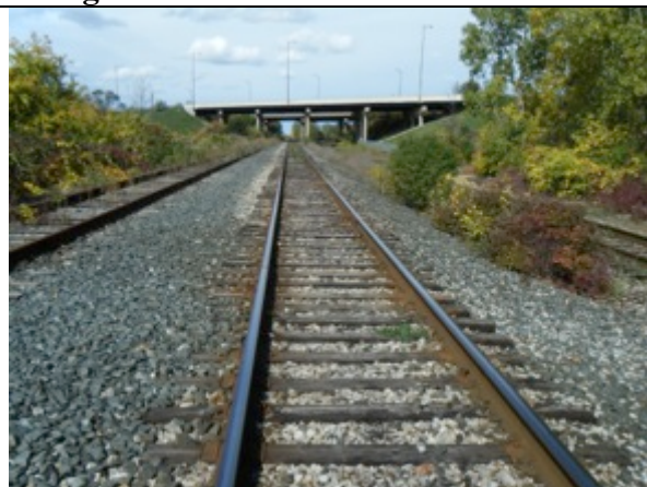
Plate 17 Railway Corridor facing northwest
