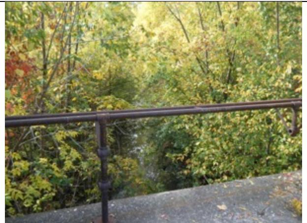
Plate 20 Drain Channel facing southwest
