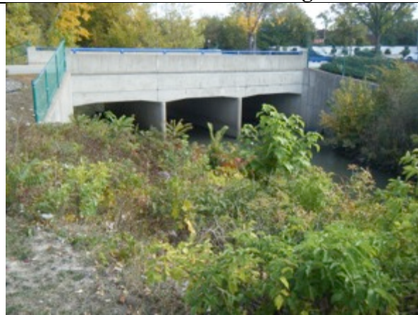
Plate 27 Plaza Parking Lot Bridge facing northeast
