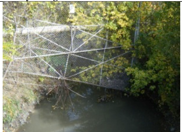
Plate 10 Drain Channel facing north
