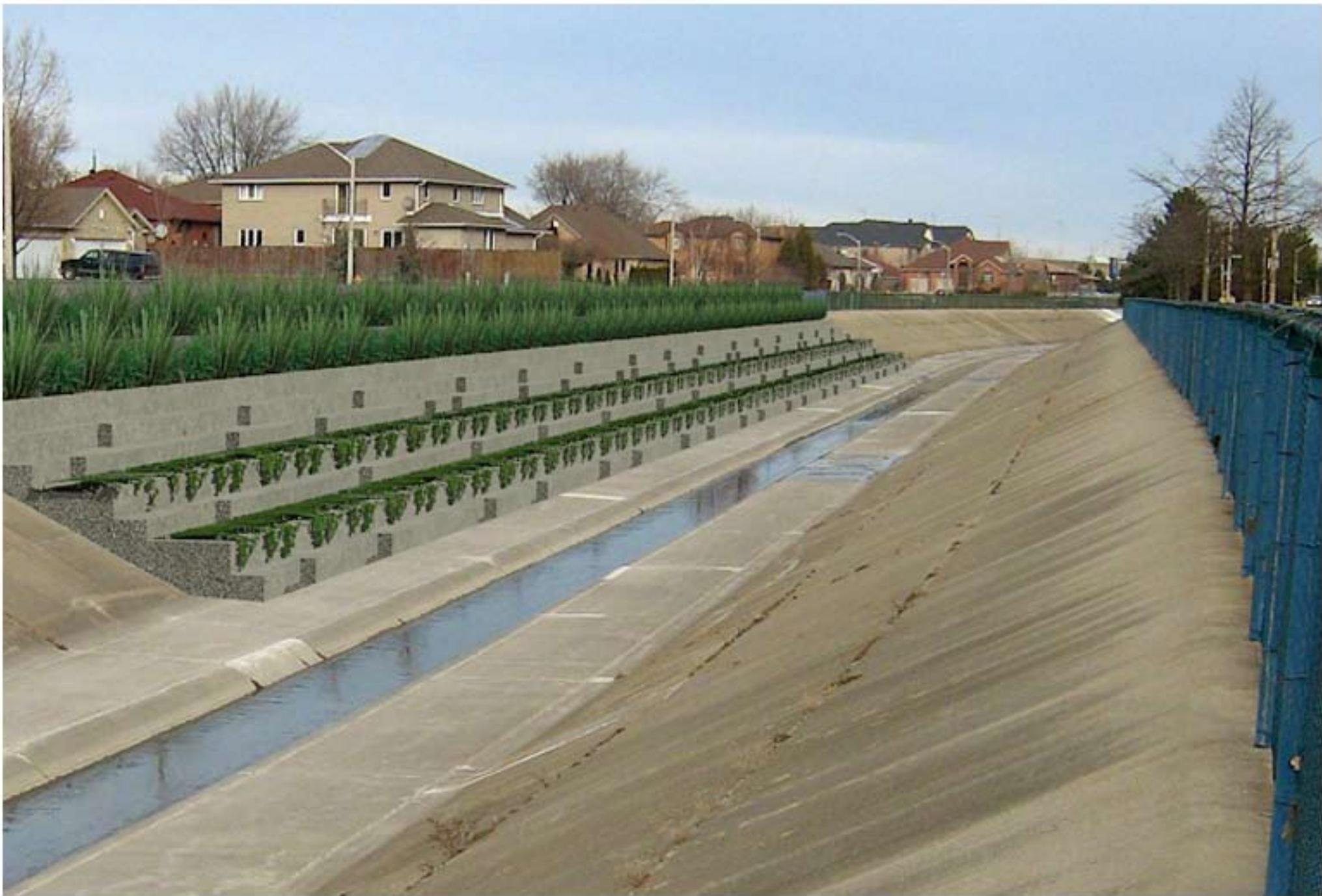
Conceptual Rendering - Option 3B - Channel Offset Stone Wall
