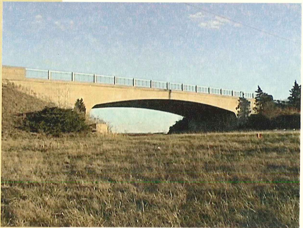
Sixth Concession Bridge at Dougall Parkway - November 1998
