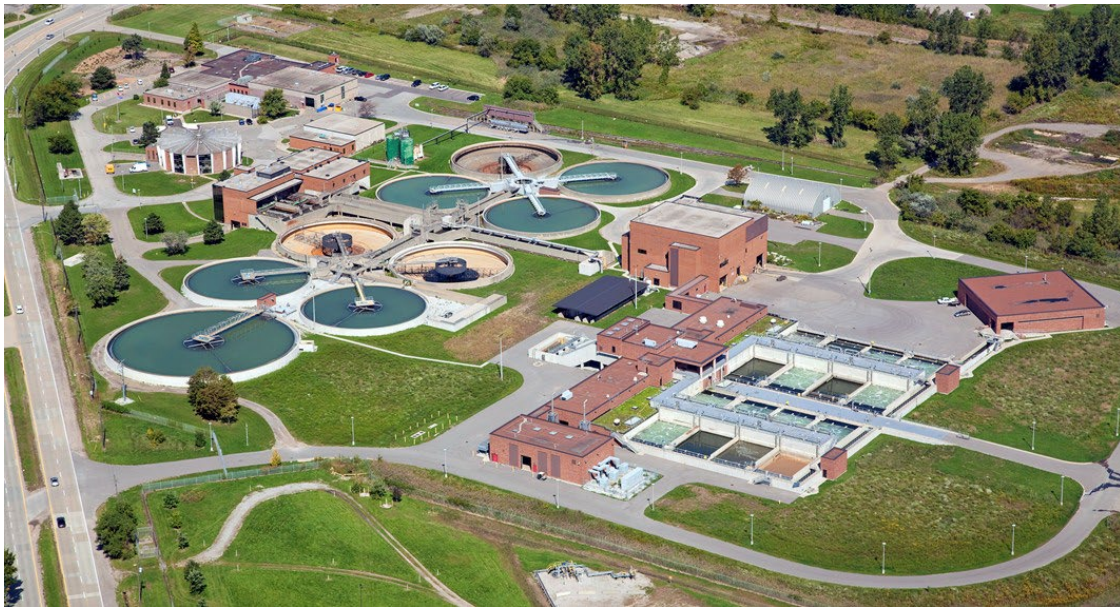
Figure 2.1: Aerial Image of the Lou Romano Water Reclamation Plant
