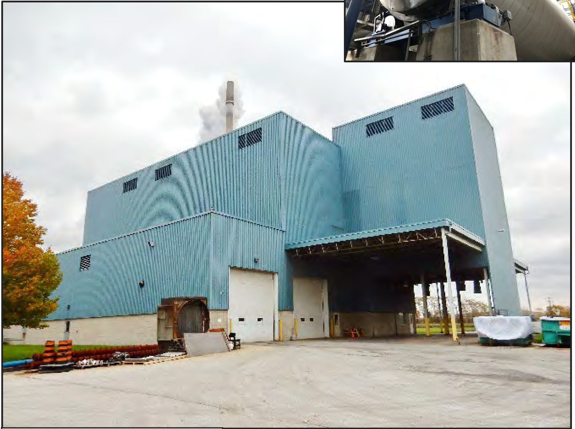
Windsor Biosolids Processing Facility
