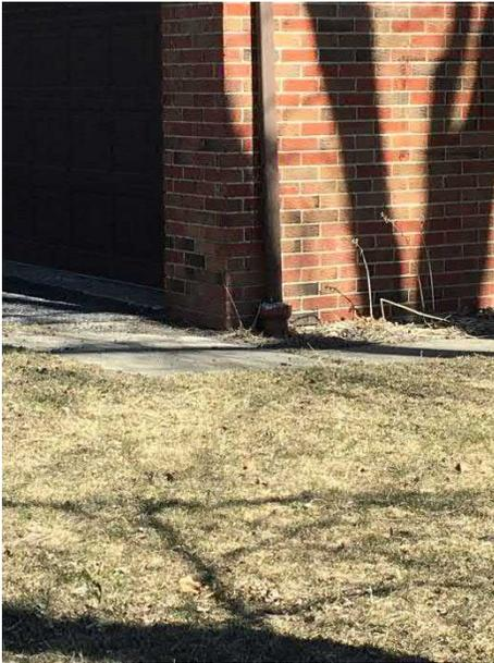
Photo 37: Connected Downspout
