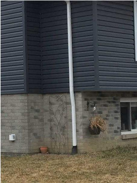
Photo 43: Connected Downspout
