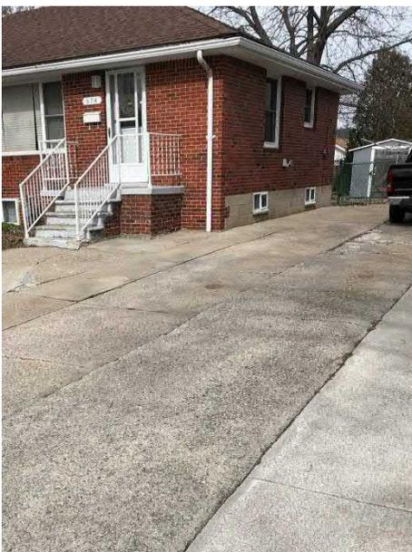
Photo 12: Connected Downspout
