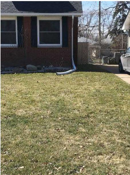
Photo 33: Disconnected Downspout
