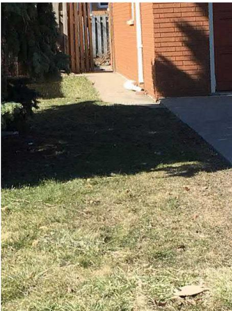
Photo 36: Disconnected Downspout
