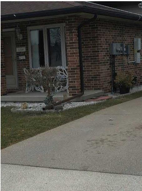
Photo 45: Disconnected Downspout
