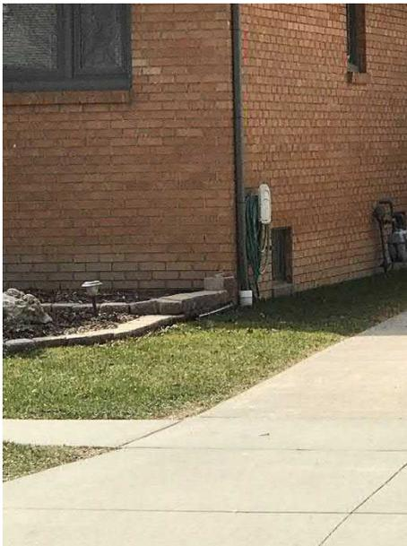
Photo 24: Connected Downspout
