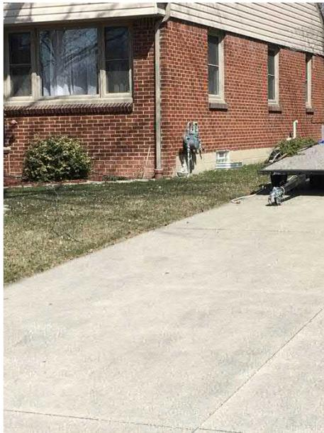
Photo 49: Connected Downspout
