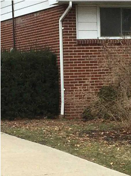
Photo 46: Connected Downspout
