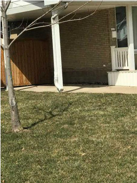
Photo 13: Disconnected Downspout
