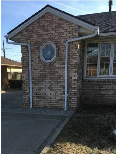
Photo 40: Connected Downspout
