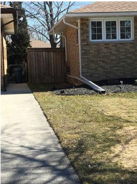
Photo 39: Disconnected Downspout
