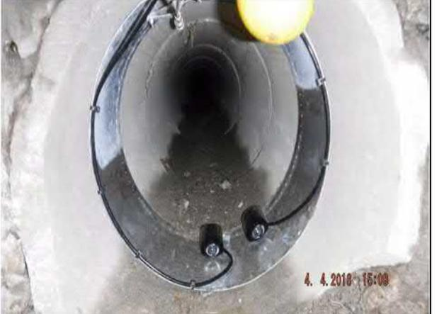
A close-up view of the flow monitor sensors installed in the manhole. The sensors are black and mounted on a metal frame. A yellow float is visible above the sensors. A timestamp in the bottom right corner reads "4. 4. 2018 15:08".                     |
