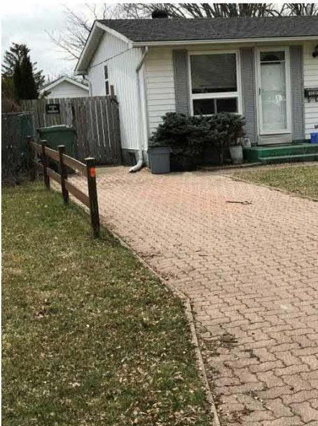
Photo 3: Disconnected Downspout
