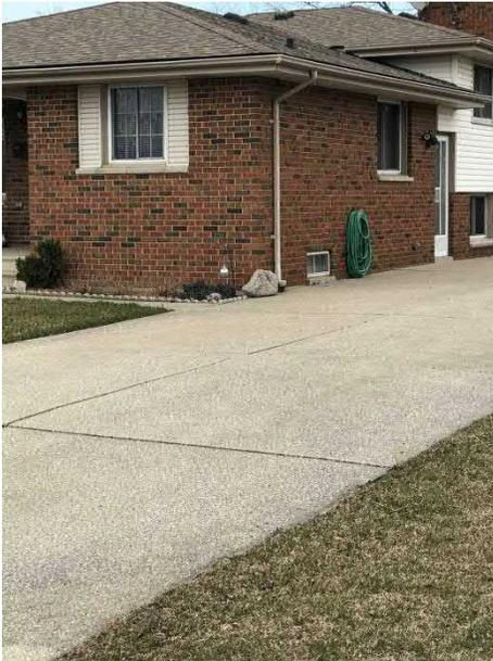
Photo 4: Connected Downspout
