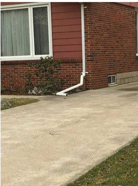
Photo 48: Disconnected Downspout
