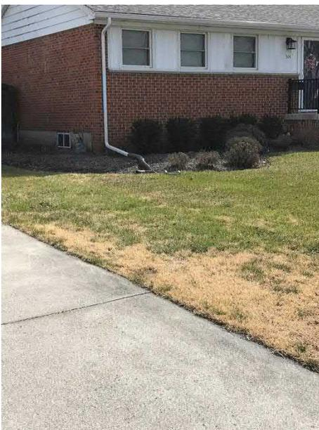
Photo 18: Disconnected Downspout
