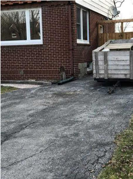
Photo 10: Disconnected Downspout
