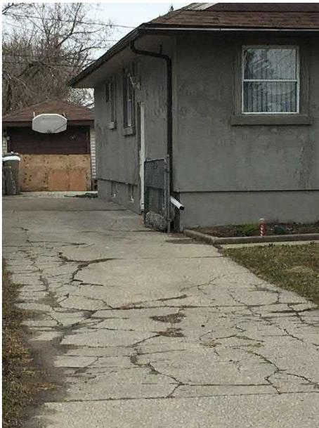
Photo 30: Disconnected Downspout
