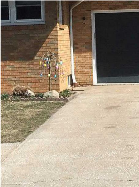
Photo 31: Connected Downspout
