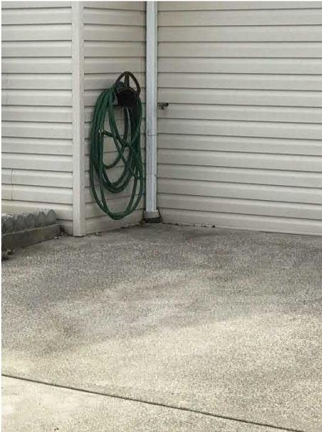
Photo 19: Connected Downspout
