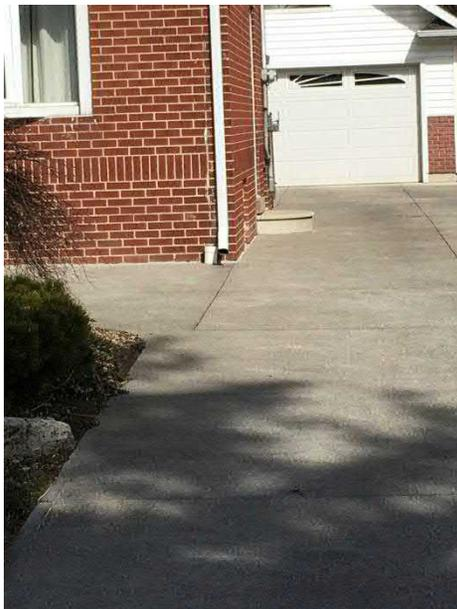
Photo 51: Disconnected Downspout
