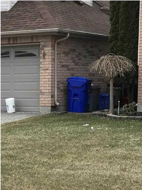
Photo 7: Disconnected Downspout
