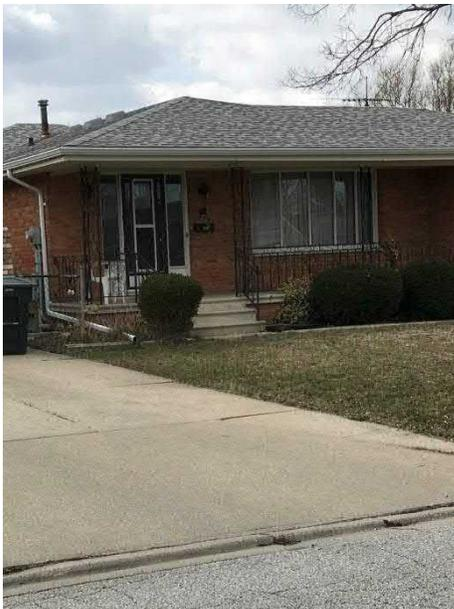
Photo 6: Disconnected Downspout
