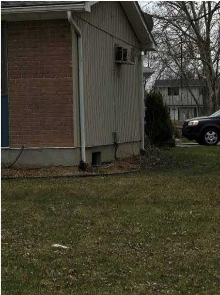
Photo 1: Connected Downspout
