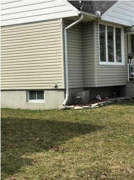
Photo 22: Disconnected Downspout
