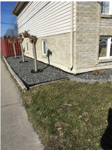
Photo 42: Disconnected Downspout
