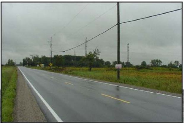
Plate 1: View to southwest showing typical disturbed ROW.
