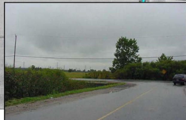
Plate 3: View to west along Intersection Road. Vegetation at left & across Banwell Rd associated with channelized stream.
