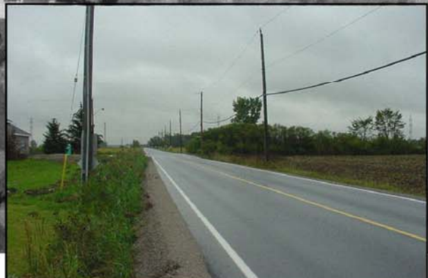
Plate 4: View to south, vegetation at right is along channelized stream. Residences at left. Note narrow elevated shoulder.
