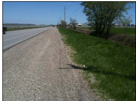
Plate 18: County Road 42 facing east, note disturbance due to ditching and roadway construction up to property line.
