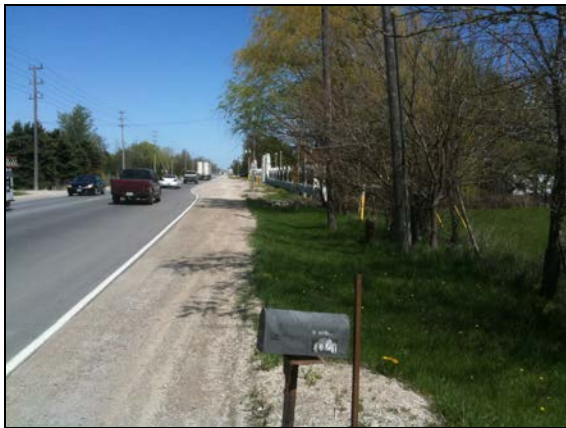
Plate 20: County Road 42 facing east, note disturbance due to ditching and roadway construction up to property line.
