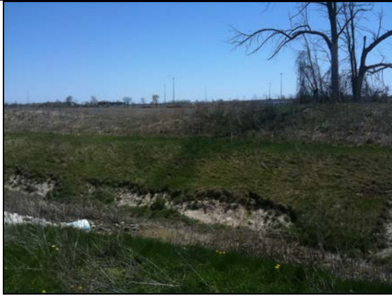
Plate 31: Walker Road, facing southeast, cultivated fields of the Future East-West Arterial from Walker Road to County Road 17.
