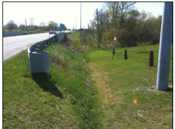
Plate 24: County Road 42 facing west, note disturbance due to ditching and services up to property line.
