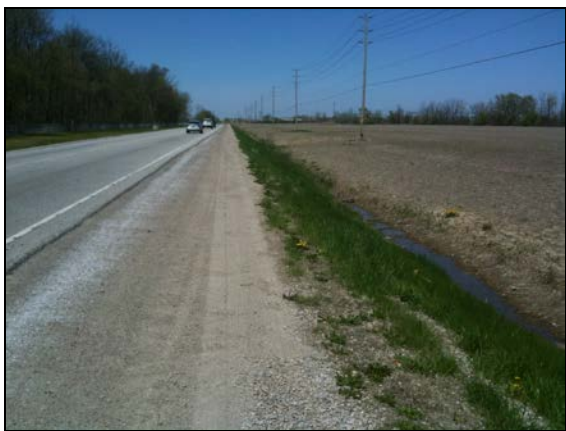
Plate 9: Lauzon Parkway facing north.
