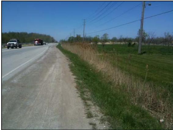
Plate 8: Lauzon Parkway facing north.
