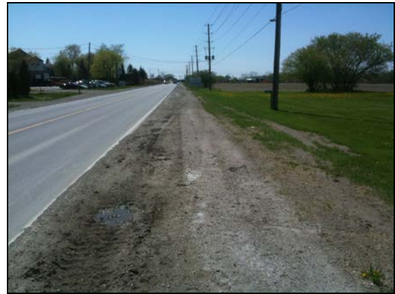
Plate 28: County Road 42 facing west, note disturbance due to roadway construction up to property line.
