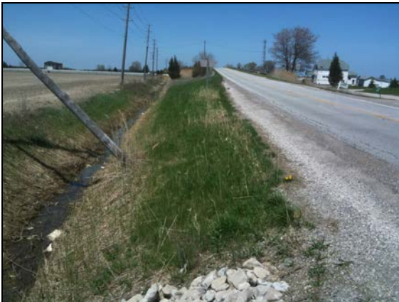
Plate 3: County Road 17 facing south, note disturbance due to ditching up to property line.
