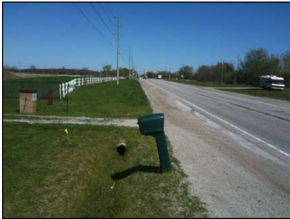
Plate 25: County Road 42 facing east, note disturbance due to ditching and services up to property line.
