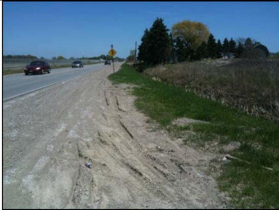
Plate 19: County Road 42 facing east, note disturbance due to ditching and roadway construction up to property line
