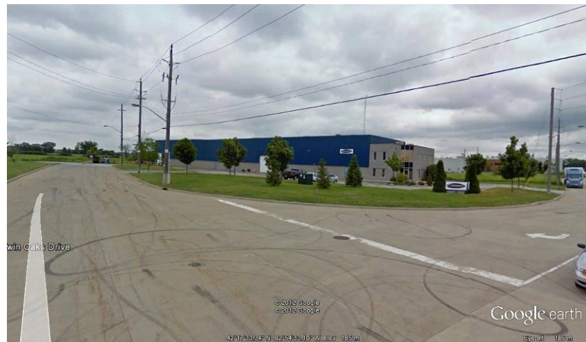
Image 4: Looking southeast at existing building and paved and landscaped areas within 9655 Twin Oaks Drive.
