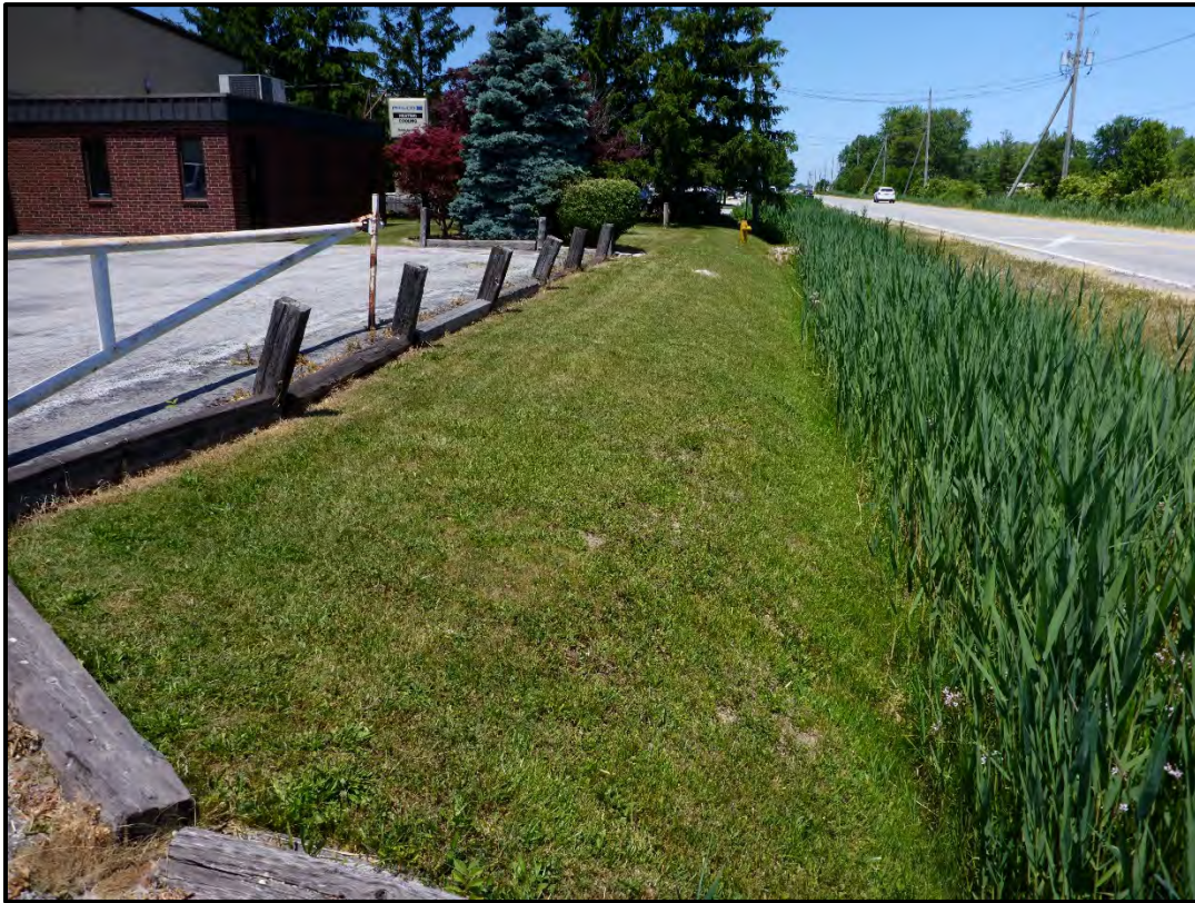
Plate 5: View of ditch along 7 th Concession Road. Facing North. June 17, 2020.
