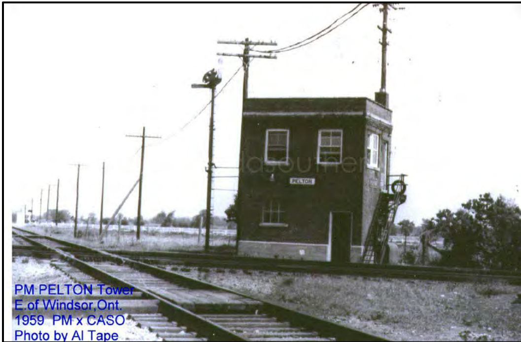
Plate 1: Pelton Tower in 1959 prior to demolition. Photo by Al Tape via Ontario Railway Maps Collection.
