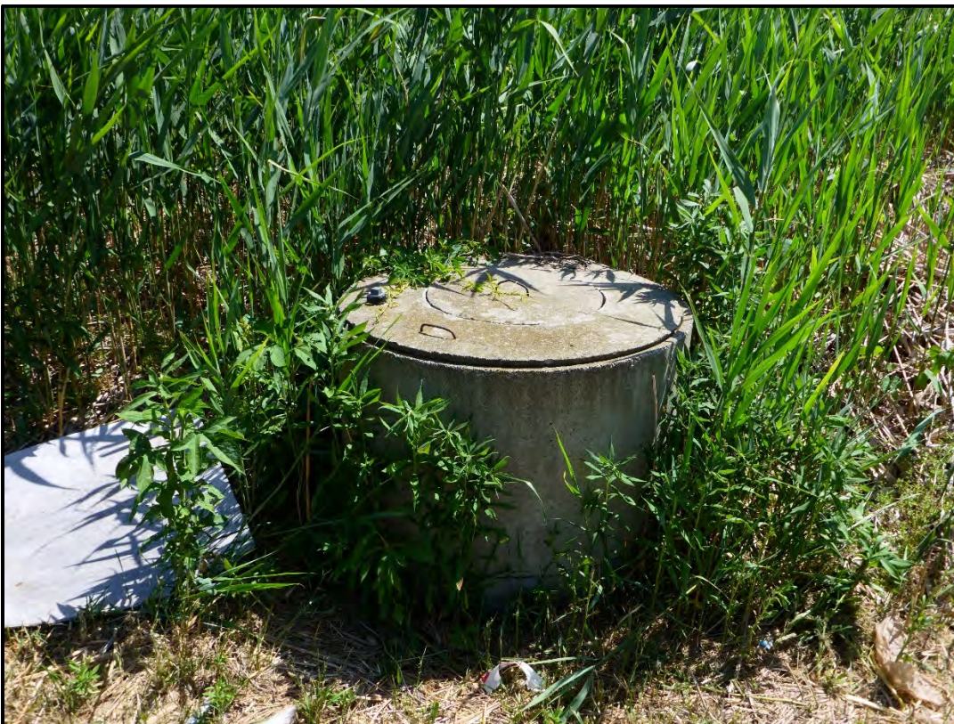
Plate 16: Septic tank manhole. Facing south. June 18, 2020.
