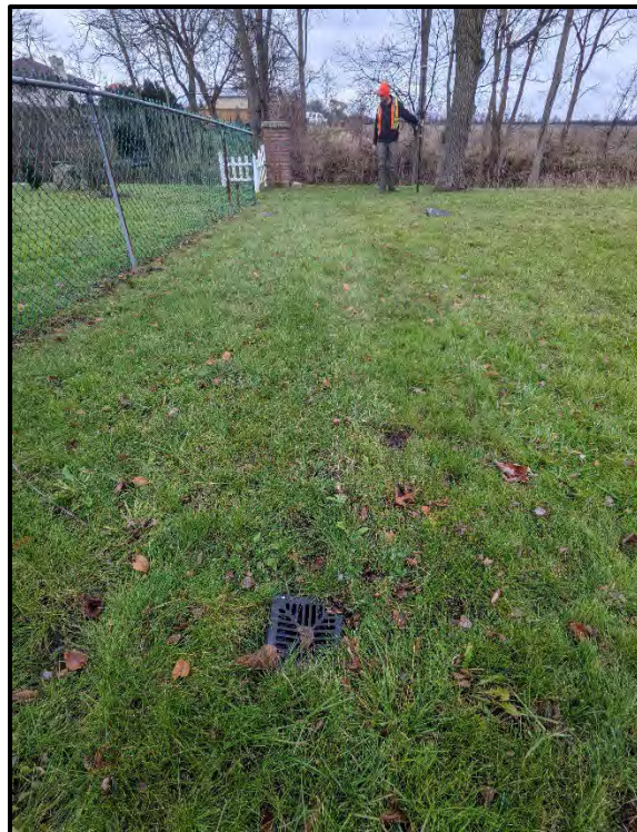
Plate 10: Drainage visible extending through the locations of several of the identified burial plots. Facing south; December 3, 2021.
