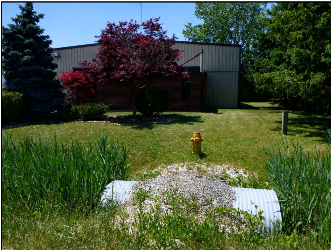
Plate 6: Ditch, culvert, and hydrant within study area along 7 th Concession Road. Facing west. June 17, 2020.
