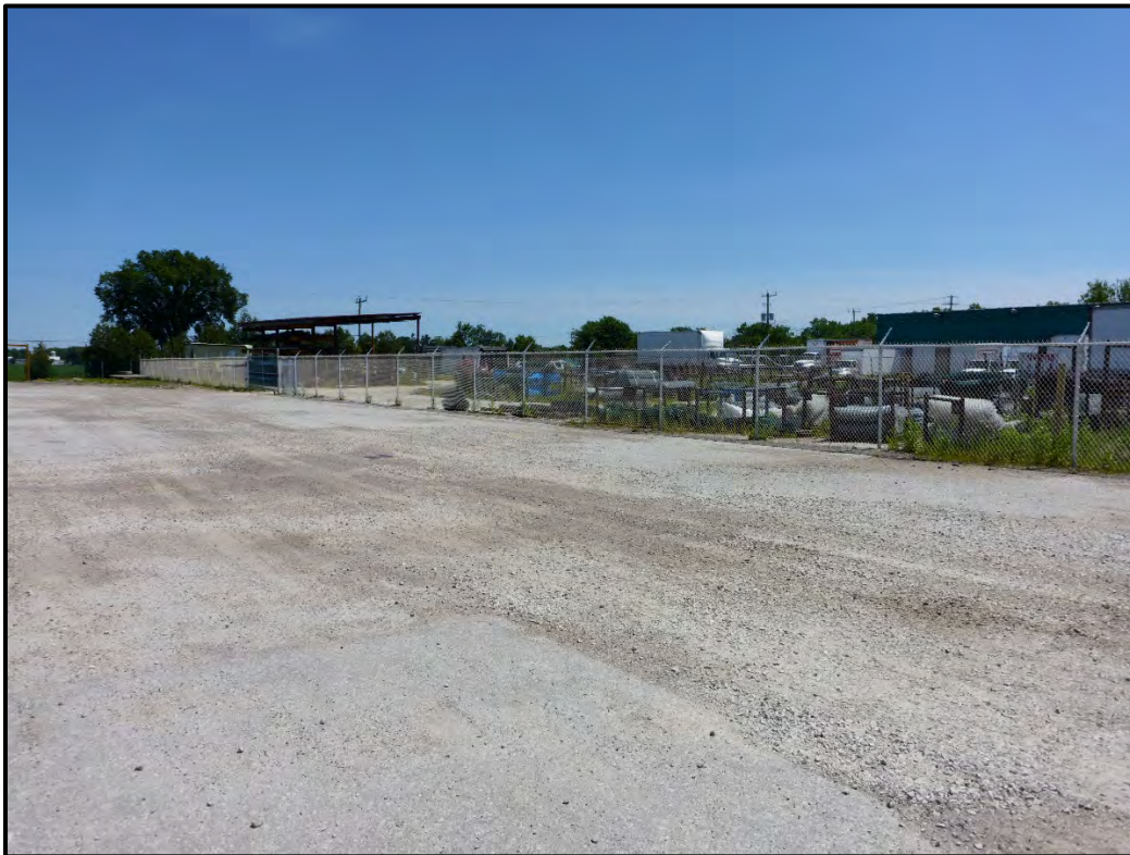
Plate 24: Parking lot and storage area. Note storm drain. Facing southeast. June 17, 2020.
