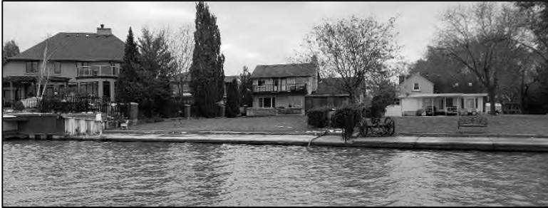
PROPERTY 69 (11906 Riverside Dr. E.) WATECH STATION 0+075 TO 0+090
