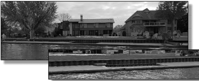
PROPERTY 48 (11600 Riverside Dr. E.) WATECH STATION 0+435 TO 0+470
